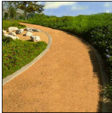
Decomposed granite surface
