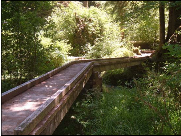
Boardwalk with low guard rails
