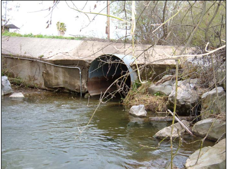
Figure 12. Fish Passage Barrier – Cecchetti Road Culvert
