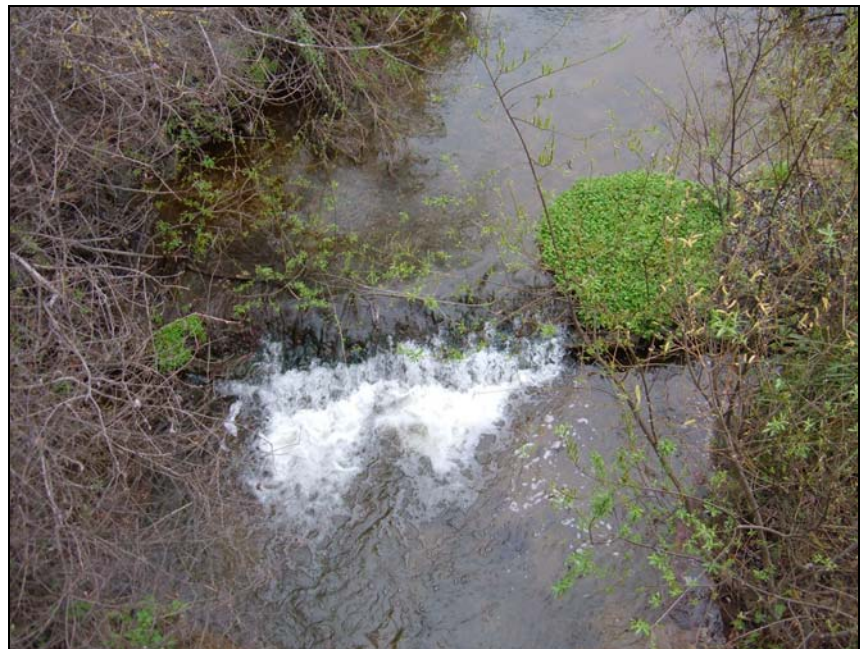
Figure 15. Fish Passage Barrier – Concrete Grade Control Weir
