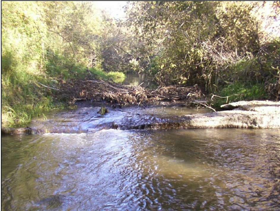
Figure 10. Fish Passage Barrier - Two Concrete Dams
