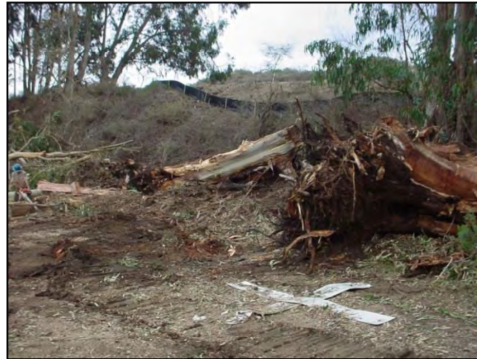
Figure 180. Silt fence from WRP violation site across Warden Creek can be seen in the distance.
