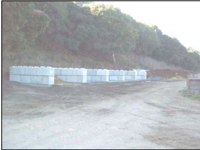
Figure 195. Blocks creating 5-bin compost facility.
