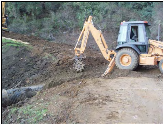
Figure 157. Compacting fill over new culvert
