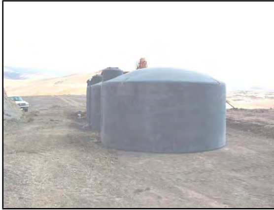
Figure 224. Three 5,000 gallon tanks on hill.
