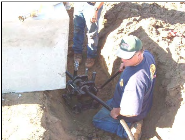
Figure 245. Installing tee to trough #30 with fusion welder.
