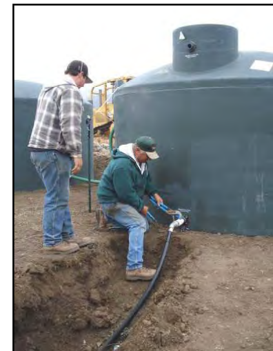
Figure 247. Tank install on south side of creek.
