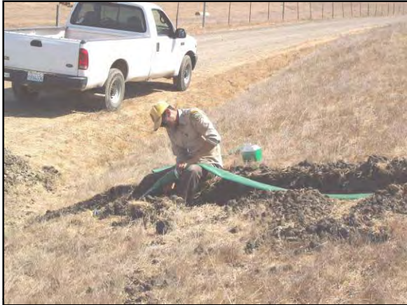
Figure 223. CCC crew leader installing 4" dia. Lay flat hose main line.
