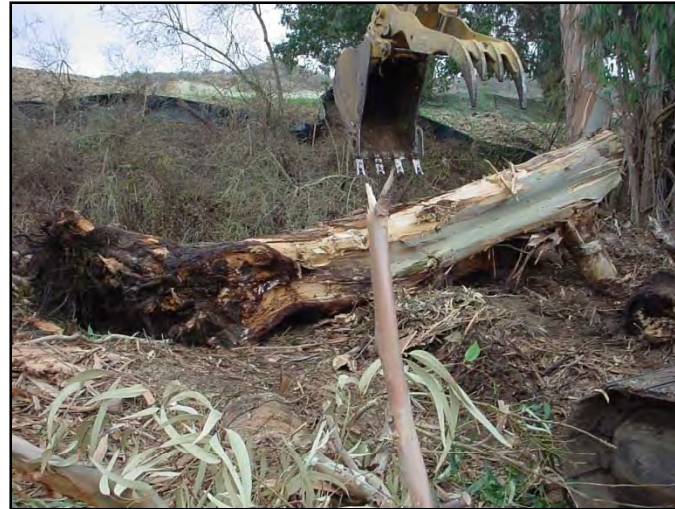
Figure 184. Root wad lifted with excavator bucket to field to be bucked up, once it was lifted out of creek.
