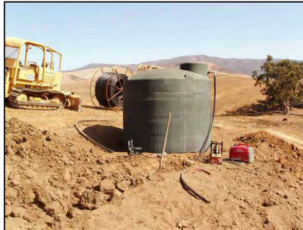
Figure 210. Installation of storage tank just below lower spring in pasture 1.
