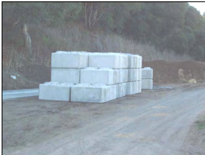
Figure 193. Inter-lock blocks off-loaded from truck, prior to placement on pad.
