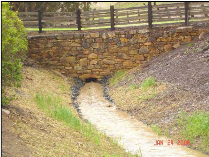
Figure 170. Looking upstream at outlet under stone bridge. Revegetated slopes are sprouting.
