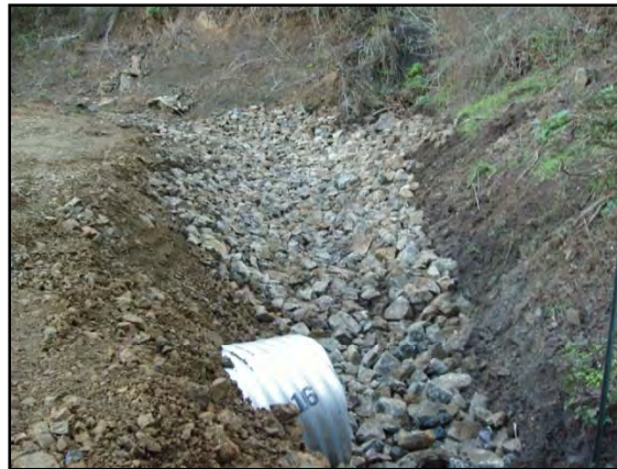
Figure 158. Improved entrance to new culvert.
