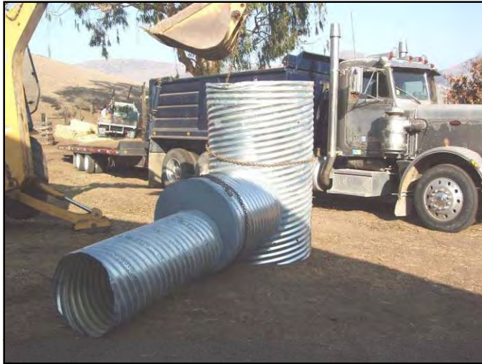
Figure 165. Drop structure prior to placement.
