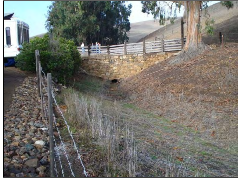
Figure 173. Looking upstream at outlet and recontoured/revegetated banks.
