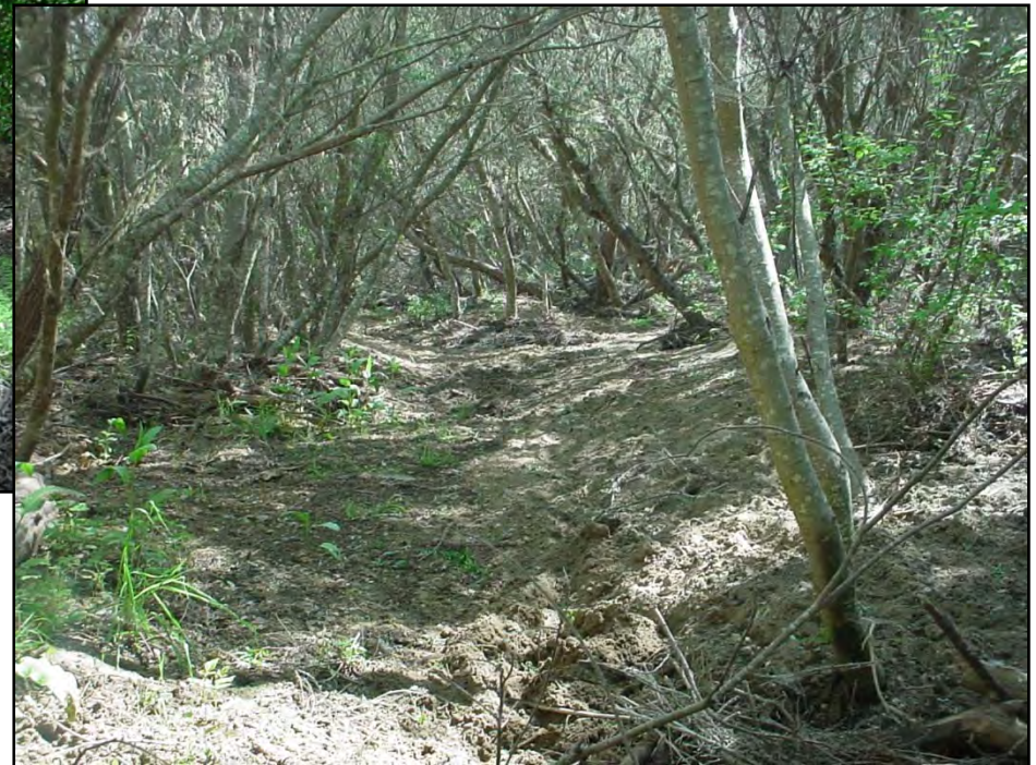
Figure 232. The channel, though clear, did catch a great deal of sediment in the 07-08 rainy season.
