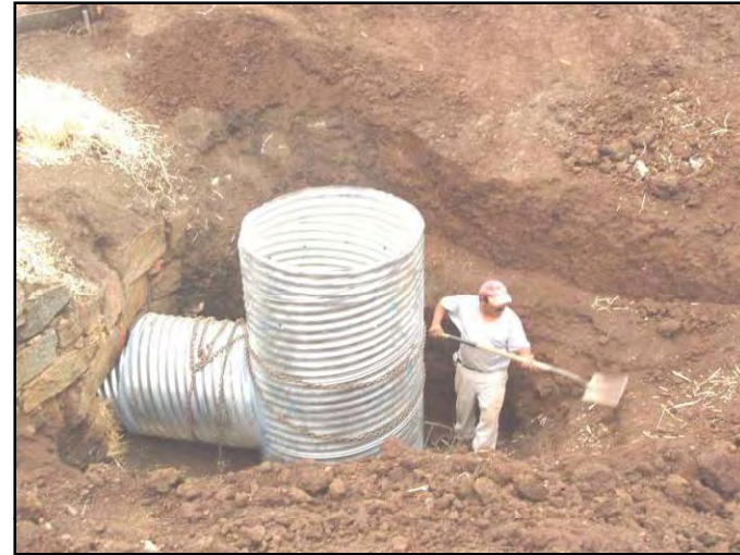
Figure 166. Placed drop structure.
