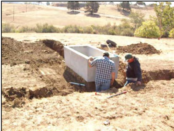
Figure 209. Installation of trough in pasture 5A.
