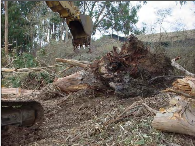
Figure 183. Root wad lifted with chain and excavator out of creek.
