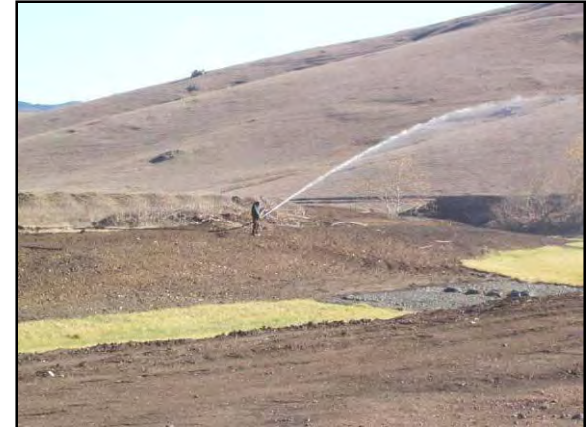
Figure 225. Cleaning rocks out of pipe.
