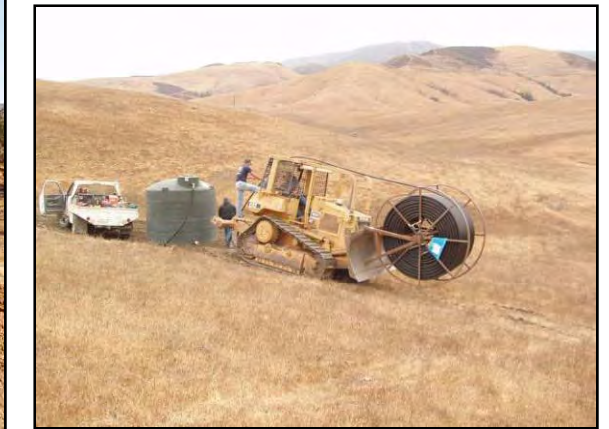
Figure 211. Installation of storage tank and pipeline to troughs in pasture 4.
