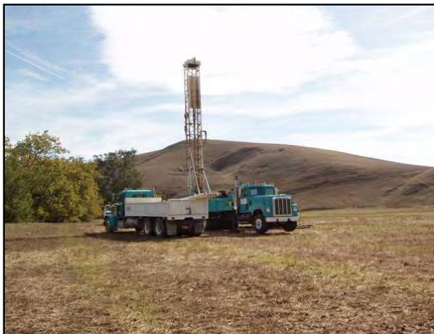
Figure 246. Site 1 well installation.
