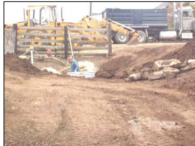
Figure 168. Headcut backfilled.
