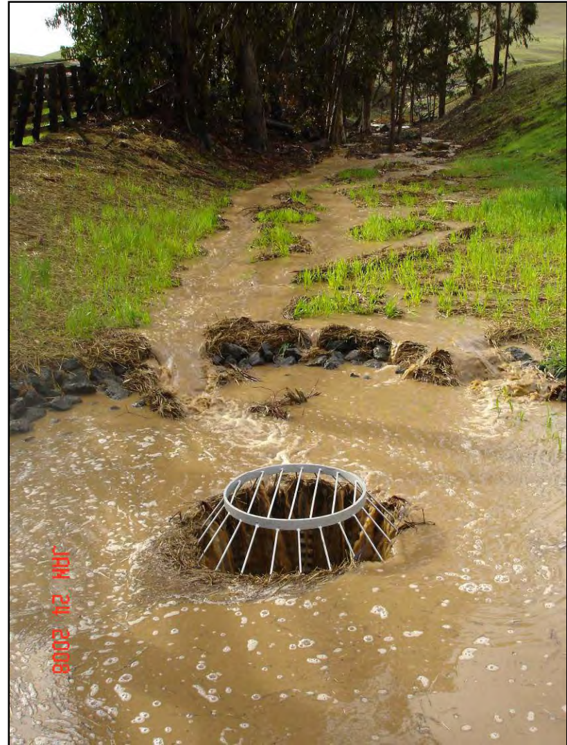
Figure 171. Looking upstream at drop structure and restored headcut during storm.
