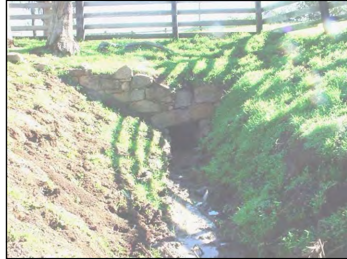
Figure 161. Looking downstream at entrance of existing rock culvert.
