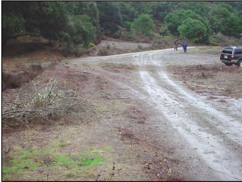
Figure 174. Road in need of repair.
