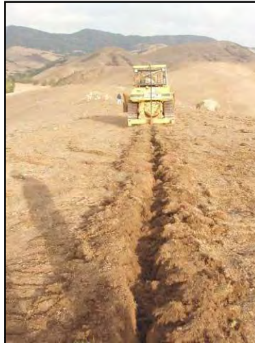
Figure 243. Ripping in pipe.
