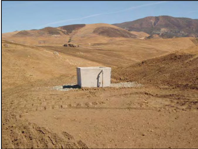
Figure 212. Trough supplied from lower fire hydrant in field 5A.
