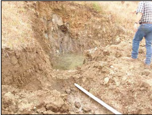
Figure 206. Development of upper spring in pasture 1.
