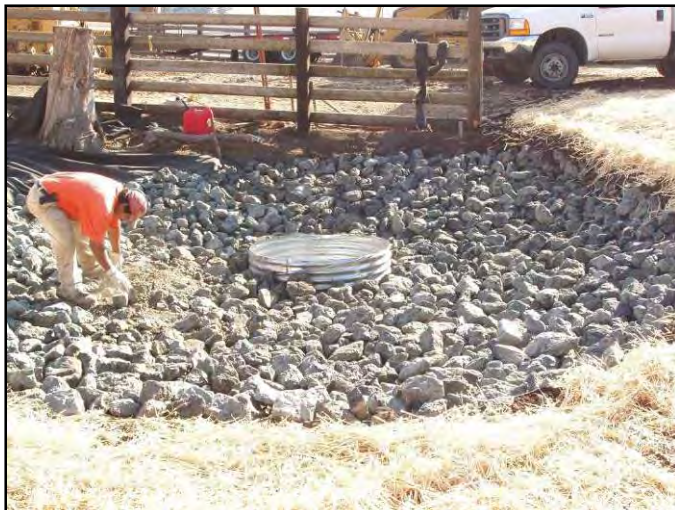
Figure 167. Looking downstream at riprap around drop.
