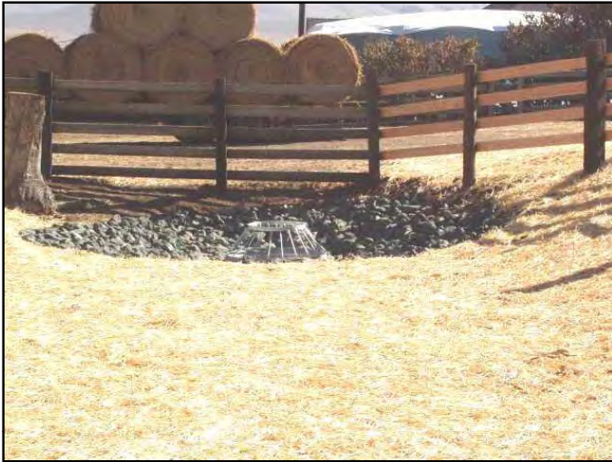
Figure 169. Installed drop structure and grate.
