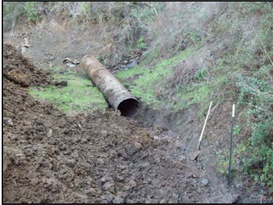
Figure 154. Failed culvert.
