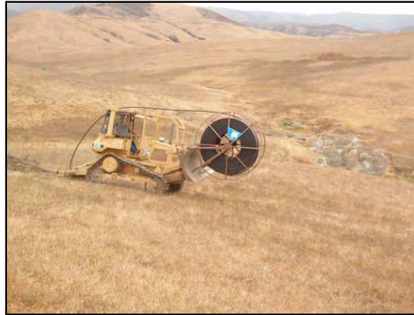
Figure 207. Ripping pipe in from upper spring in pasture 1 to trough.
