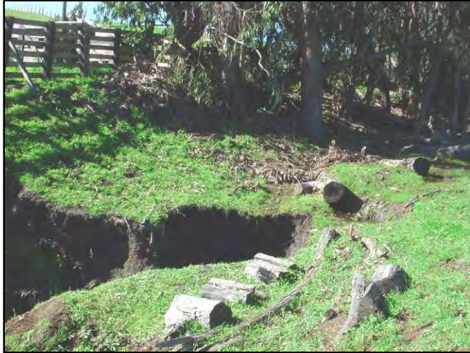
Figure 160. View of headcut, looking from left bank to right bank.
