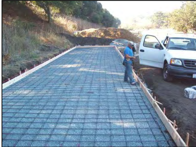
Figure 191. Contractor tying steel for pad.
