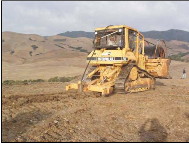
Figure 242. Cat and spool system used to rip in pipe.
