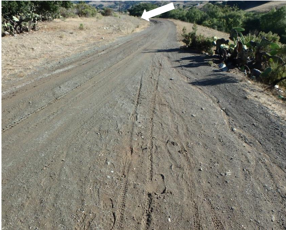
Photo 107. Site 238.1 (Stenner Creek Rd.): View of Site 238.1 looking towards Site 238 (see arrow). Evidence of poor road drainage is visible to the evidenced by presence of rilling from concentrated road runoff. Mainstem Stenner Creek runs parallel to this road on the right side of the frame.
