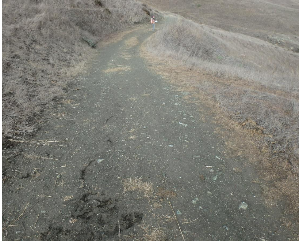
Photo 9. Site 195.2 (Powerline Rd.): View of Site 195.2 looking up the road at an unstable road fillslope. This section of road is located at the headwaters of a Class III stream. The steep fillslope is saturated and has the potential for failure.
