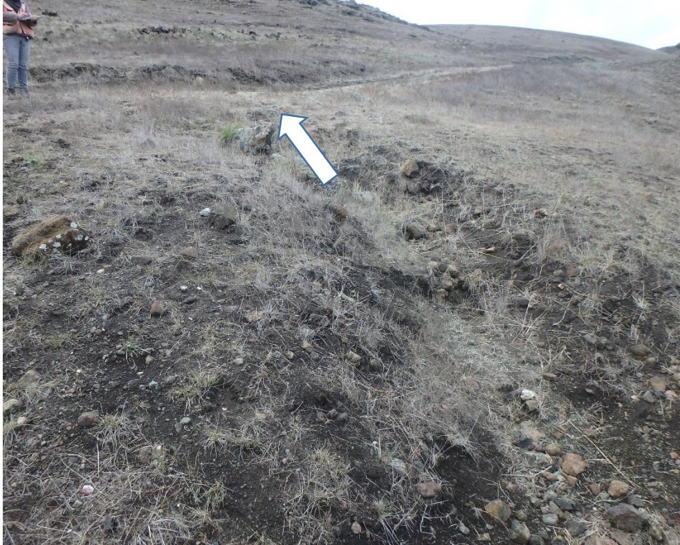
Photo 11. Site 195.3 (Powerline Rd.): View of Site 195.3 looking up at the road surface discharge point and subsequent gully (see arrow). Nearly 450' of road and hillslope runoff exit the road at this location.
