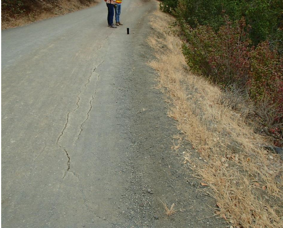
Photo 95. Site 232.1 (Poly Canyon Rd.): View of Site 232.1 looking southwest. Site 232.1 is located above mainstem Brizziolari Creek. Tension cracks in the road indicate a potential road fill failure.
