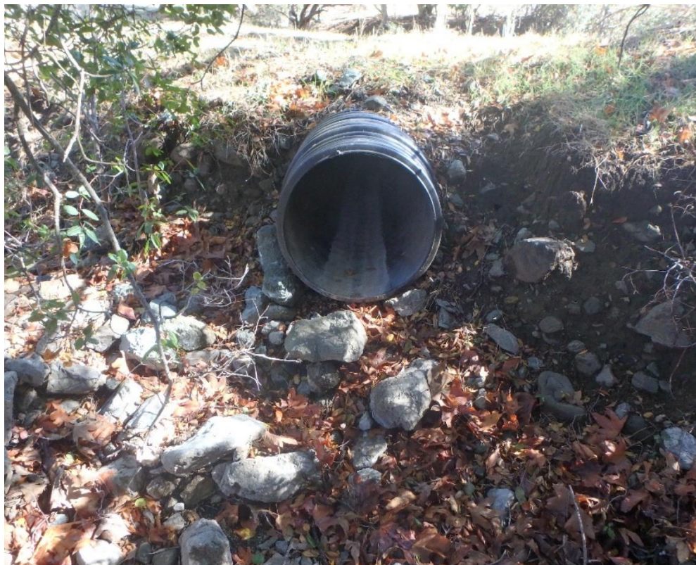
Photo 68. Site 220 (Peterson Ranch Rd.): View of Site 220 looking upstream at the culvert outlet area. Fine sediment from a recent storm is visible on the bottom of the corrugated plastic pipe.
