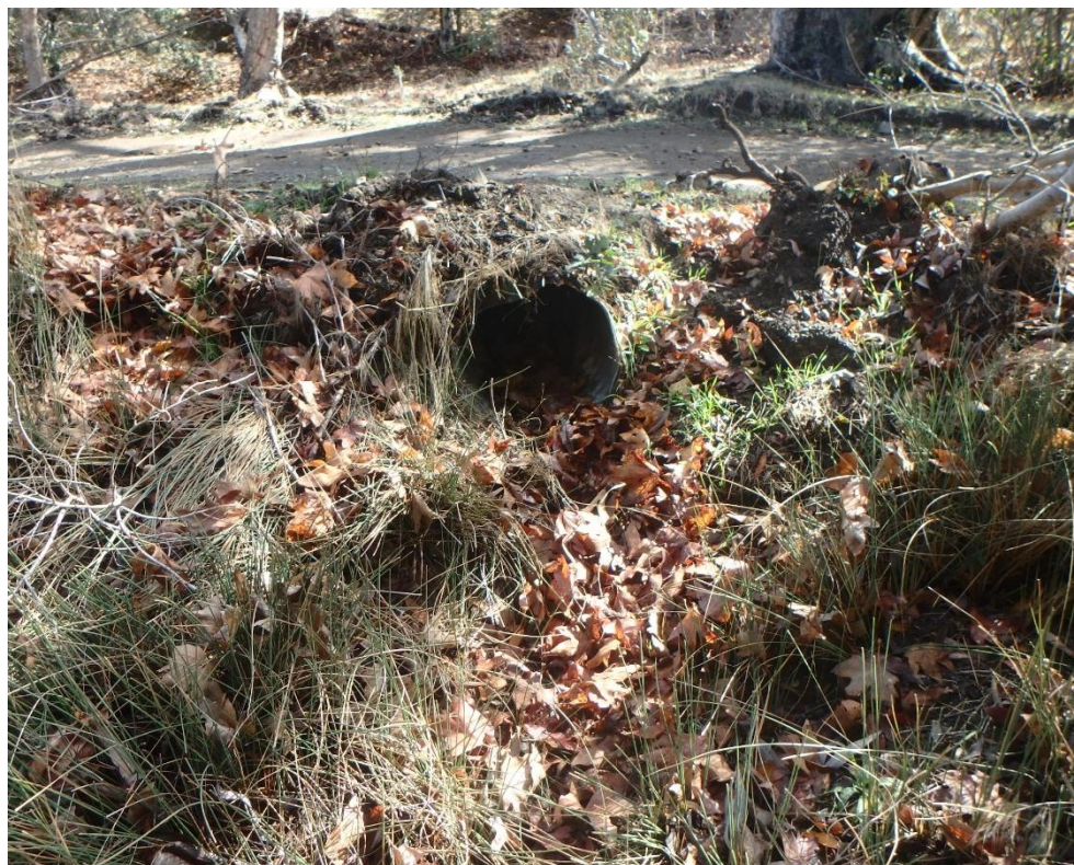
Photo 70. Site 221 (Peterson Ranch Rd.): View of Site 221 looking upstream at the culvert outlet area. This section of road runs adjacent to mainstem Brizziolari Creek and frequently becomes inundated during wet weather events.
