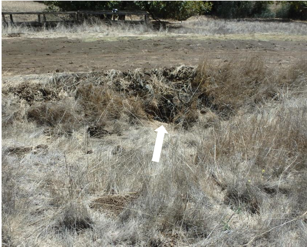
Photo 83. Site 227.1 (Peterson Ranch Rd.): View of Site 227.1 plugged ditch relief culvert inlet (see arrow) looking towards mainstem Brizziolari Creek. The road crossing is also visible in the top of the frame.
