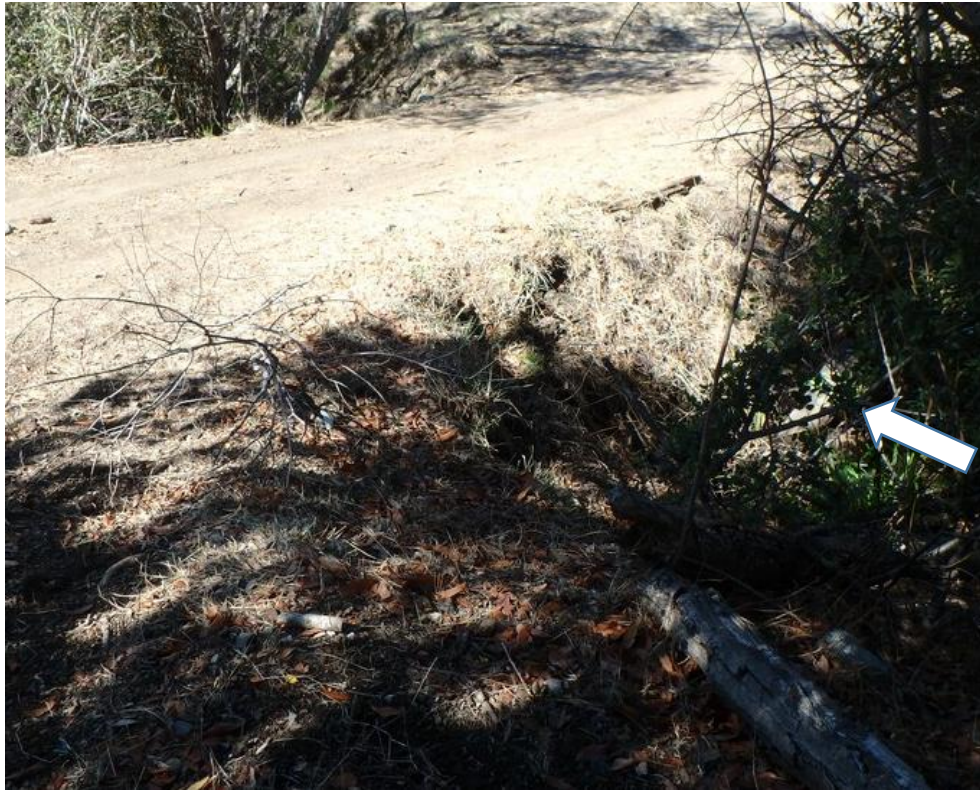
Photo 43. Site 209 (Peterson Ranch Rd.): View of Site 209 looking obliquely at the undersized stream crossing (see arrow). The right road is visible in the uppermost right frame. The stream flows from right to left.
