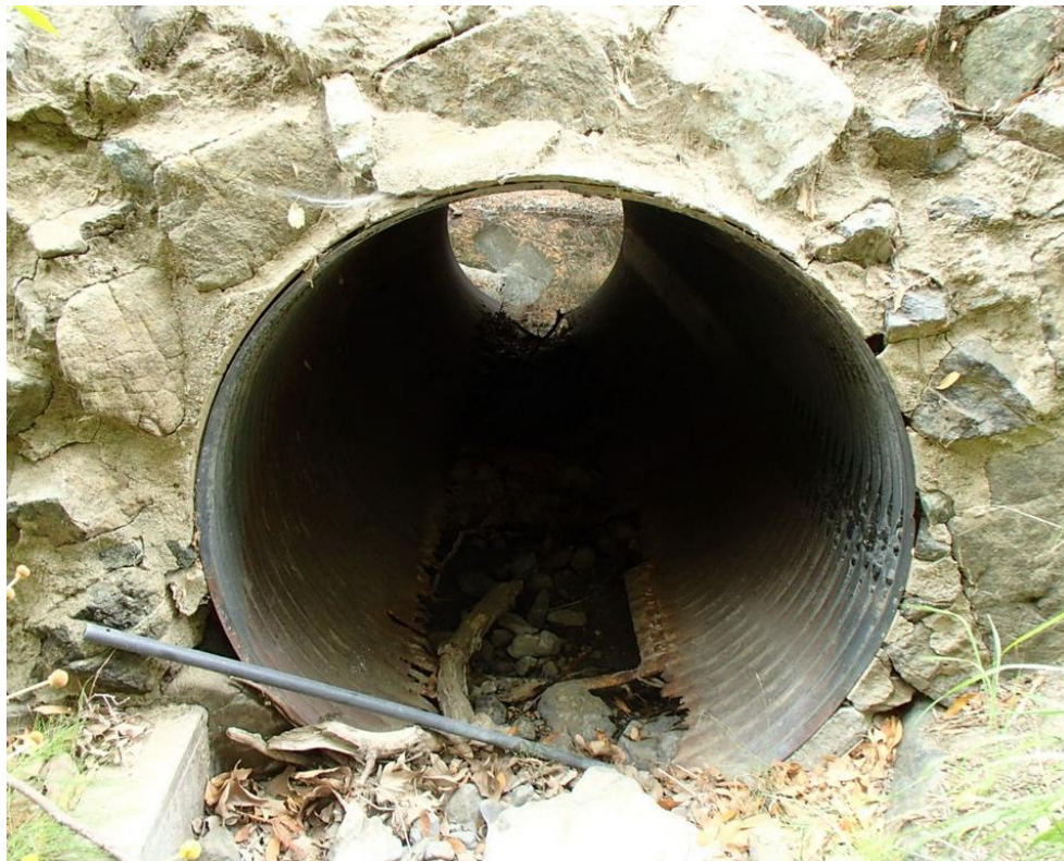
Photo 90. Site 230 (Poly Canyon Rd.): View of Site 230 culvert inlet. Looking downstream, notice the rusted-out bottom of the culvert and the washed-out trash rack.
