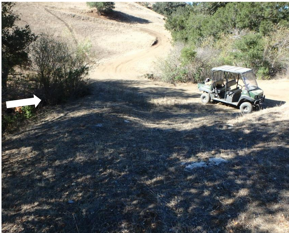
Photo 48. Site 211 (Peterson Ranch Rd.): View of Site 211 looking up the left road and obliquely at the stream crossing. The culvert inlet area is visible in the upper left frame (see arrow) and the culvert outlet area is visible in the upper right frame.
