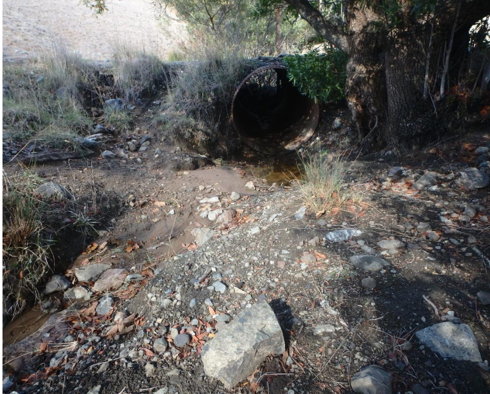
Photo 41. Site 208 (Peterson Ranch Rd.): View of Site 208 looking upstream at the culvert outlet area. Fine sediment generated from road surface erosion is visible below and to the left of the culvert outlet. The culvert is adequately sized but vertical fillslopes are eroding and unstable.
