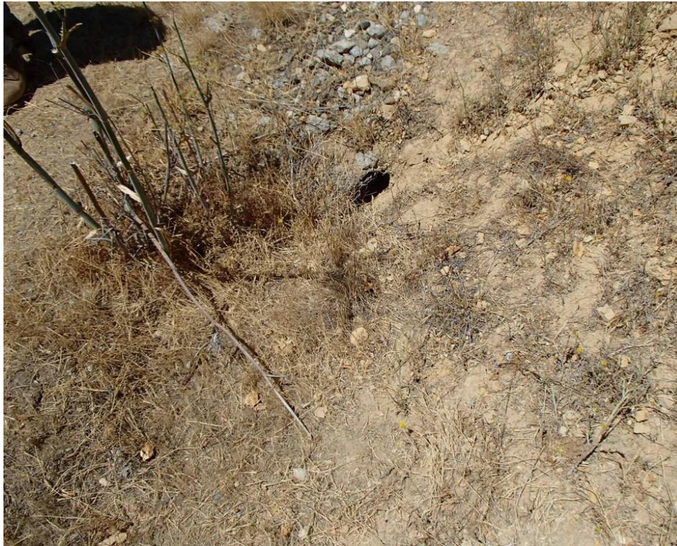
Photo 21. Site 198.1 (Barn Rd.): View of Site 198.1 looking downslope at the ditch relief culvert inlet area. The culvert inlet is approximately 50% plugged with sediment.
