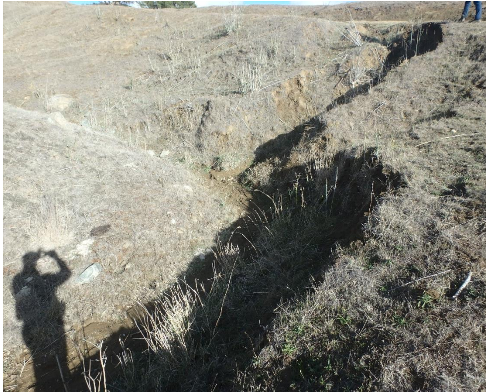
Photo 39. Site 207 (Peterson Ranch Rd.): View of Site 207 looking up at the road surface discharge point from the Class II stream. The discharge point is in the upper right corner of the frame and has created the 15' wide x 25' long erosional gully.
