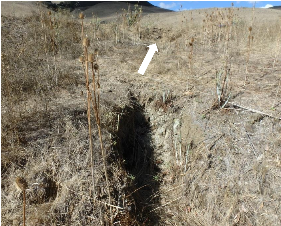
Photo 74. Site 223 (Peterson Ranch Rd.): View of Site 223 looking upstream at the culvert outlet. The outlet and the road crossing are visible in the top of the frame (see arrow) while erosion is visible in the center of the frame.
