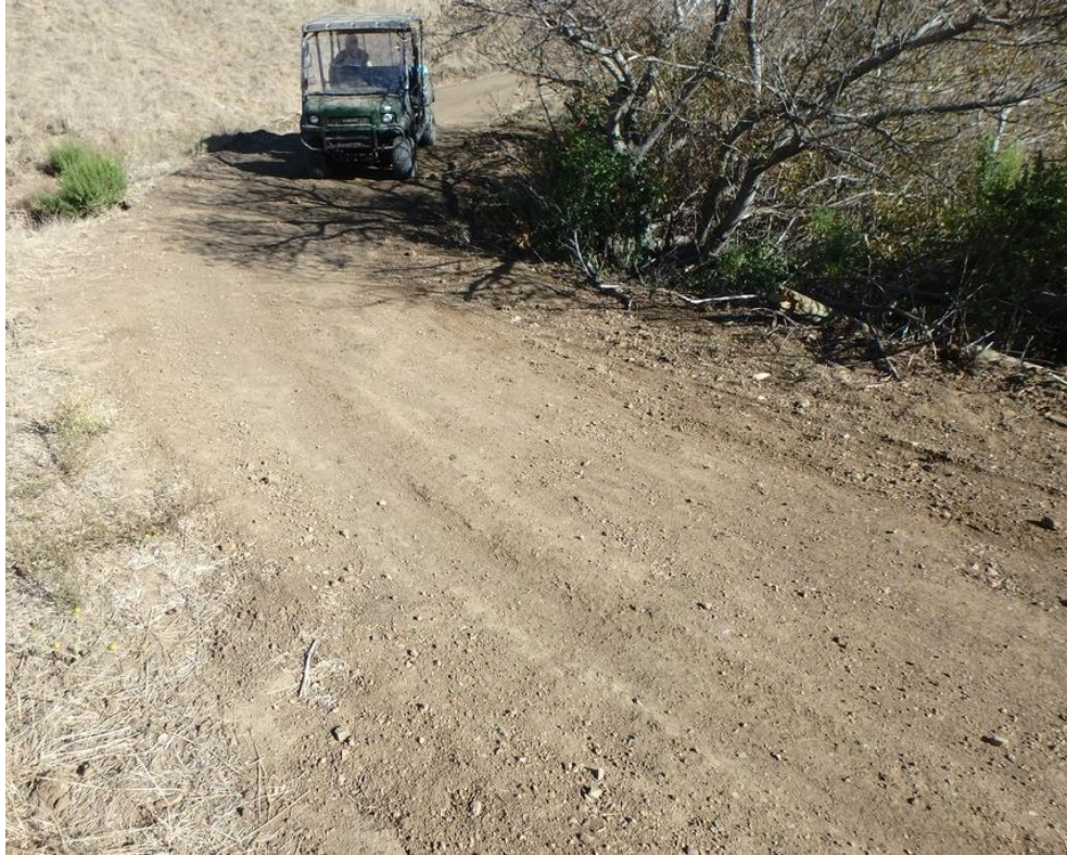
Photo 51. Site 213 (Peterson Ranch Rd.): View of Site 213 looking obliquely at the undersized stream crossing. The culvert outlet area is visible in the right frame located to the right of the ATV. The stream flows from left to right.
