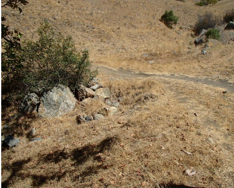
Photo 29. Site 202 (Upper Stenner Spur): View of Site 202 looking obliquely at the stream crossing. The outboard fill riprap has dislodged in this location and a gully is migrating into the trail.
