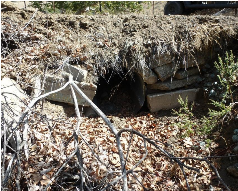
Photo 64. Site 218 (Peterson Ranch Rd.): View of Site 218 looking upstream at the culvert outlet. Some concrete block fill is visible in the center of the frame.
