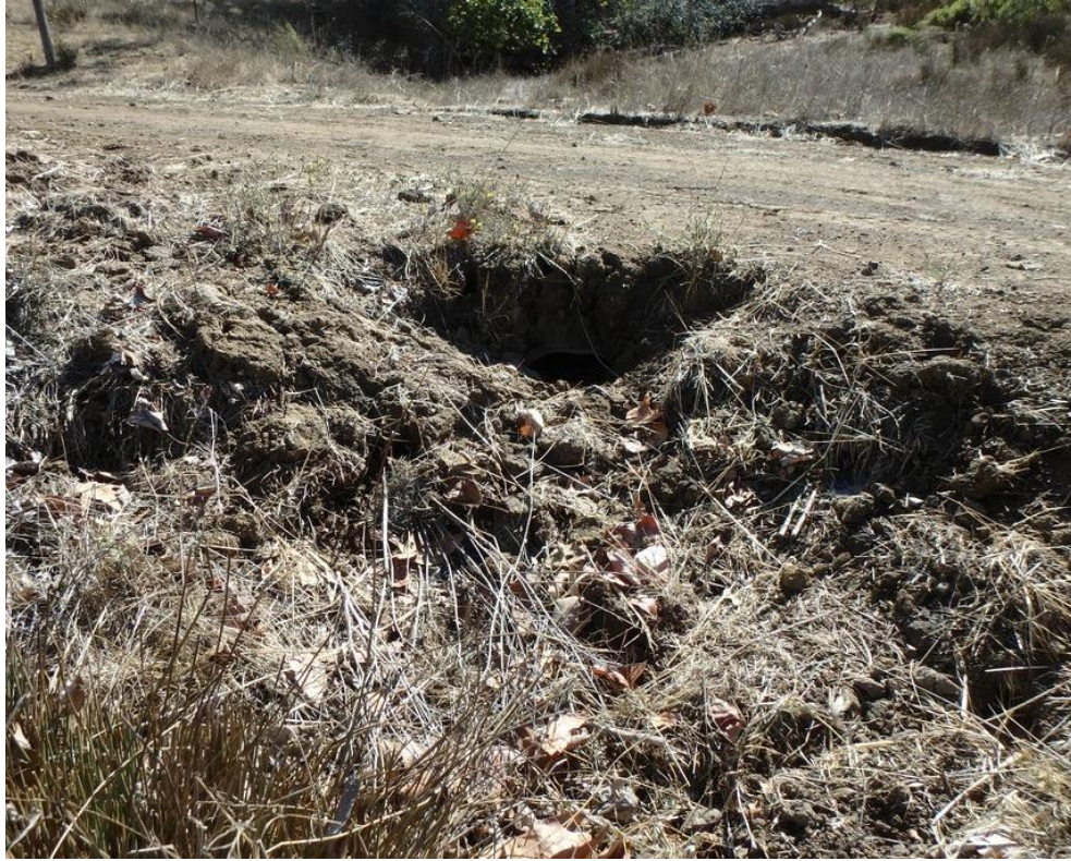
Photo 65. Site 219 (Peterson Ranch Rd.): View of Site 219 looking upstream at culvert outlet area. The plugged culvert is visible in the center of the frame.
