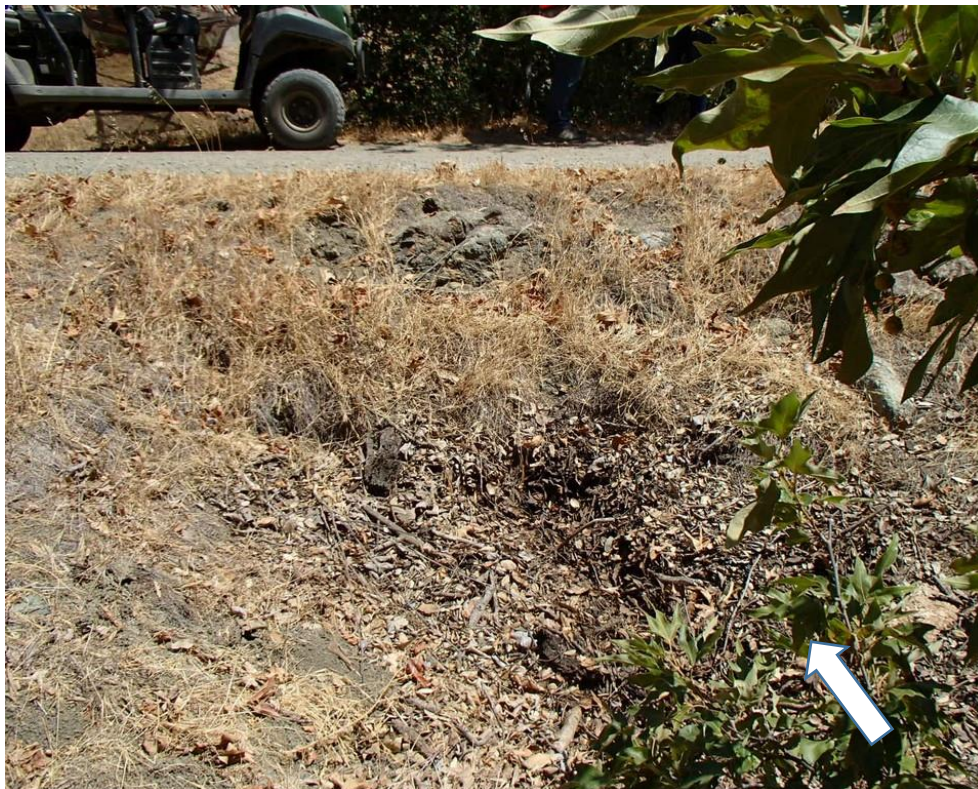
Photo 6. Site 195 (Architectural Canyon Complex Rd.): View of Site 195 looking downstream. The culvert is plugged with detritus at the center of the frame (see arrow). The road crossing is visible at the top of the frame. The stream flows from right to left.
