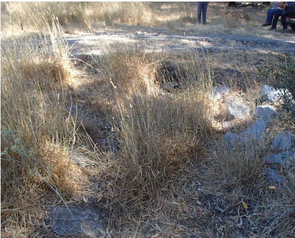
Photo 26. Site 200 (Barn Rd.): View of Site 200 ditch relief culvert outlet area. Looking upslope, the outlet is present in the center of the photo and is approximately 30% plugged.
