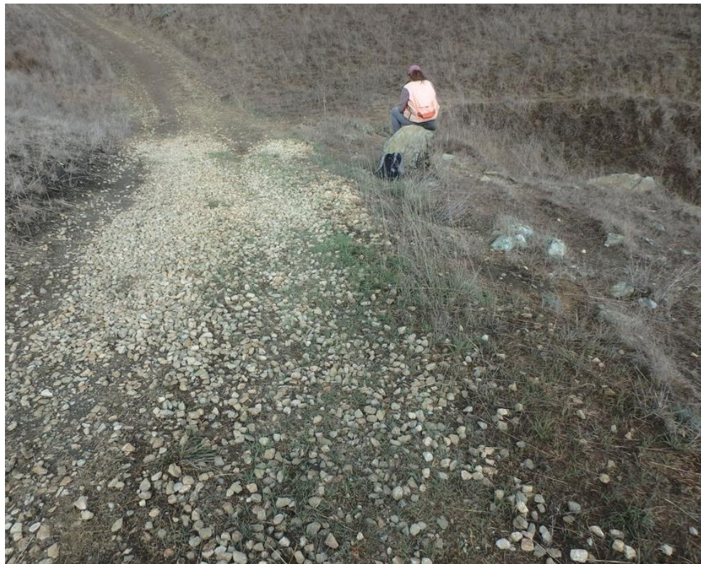
Photo 8. Site 195.1 (Powerline Rd.): View of Site 195.1 looking down the right road approach towards the stream crossing. The proximity of the headcut to the road is visible in the upper right frame. The left road approach is visible in the upper left corner of the photo.
