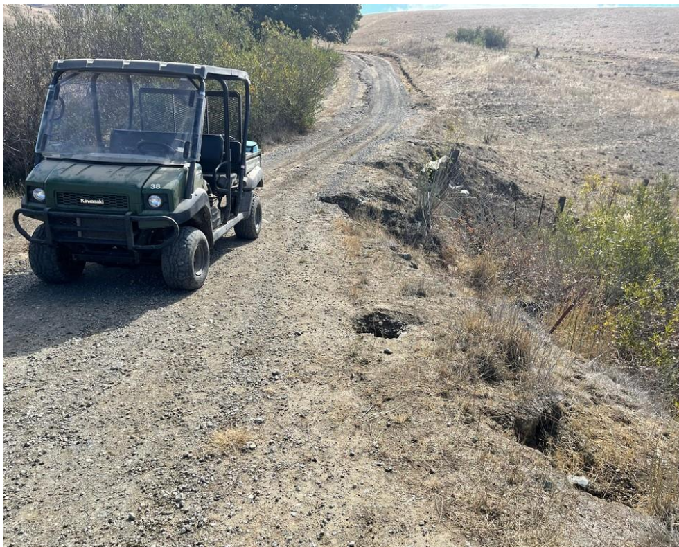
Photo 38. Site 206 (Peterson Ranch Rd.): View of Site 206 looking up left road and obliquely at stream crossing. Evidence of sediment discharge from road erosion is visible along the outboard edge of the road in the center of the frame.
