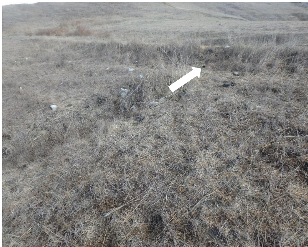
Photo 78. Site 225 (Peterson Ranch Rd.): View of Site 225 looking upslope towards the culvert outlet area (see arrow). The gully that has formed as a result of the culvert discharge is visible in the center left of the frame.
