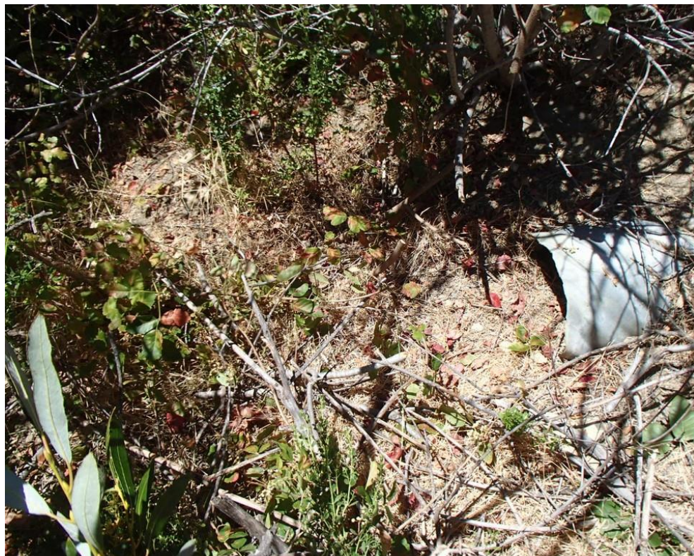
Photo 20. Site 198 (Barn Rd.): View of the ditch relief culvert outlet area at Site 198. The culvert outlet is approximately 50% plugged with sediment.
