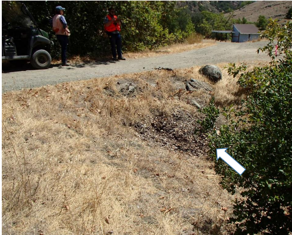
Photo 5. Site 195 (Architectural Canyon Complex Rd.): View of Site 195 looking obliquely at the stream crossing. The undersized culvert inlet is plugged with organic matter at the center of the frame (see arrow). Partial view of right approach.
