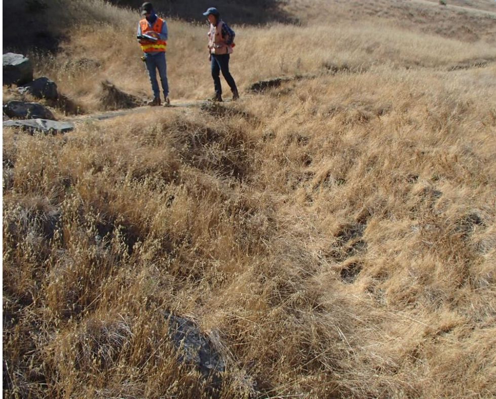
Photo 113. Site 412 (Yewks Trail): View of Site 412 looking upstream towards the stream crossing. The stream channel is grassed over, and the outboard fillslope is armored with riprap.
