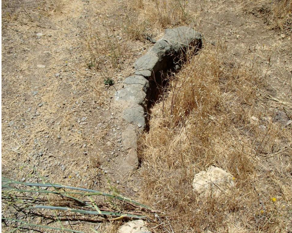
Photo 19. Site 198 (Barn Rd.): View of the ditch relief culvert inlet area at Site 198. A short rock wall encases the culvert in this location. The culvert inlet is mostly plugged with sediment.
