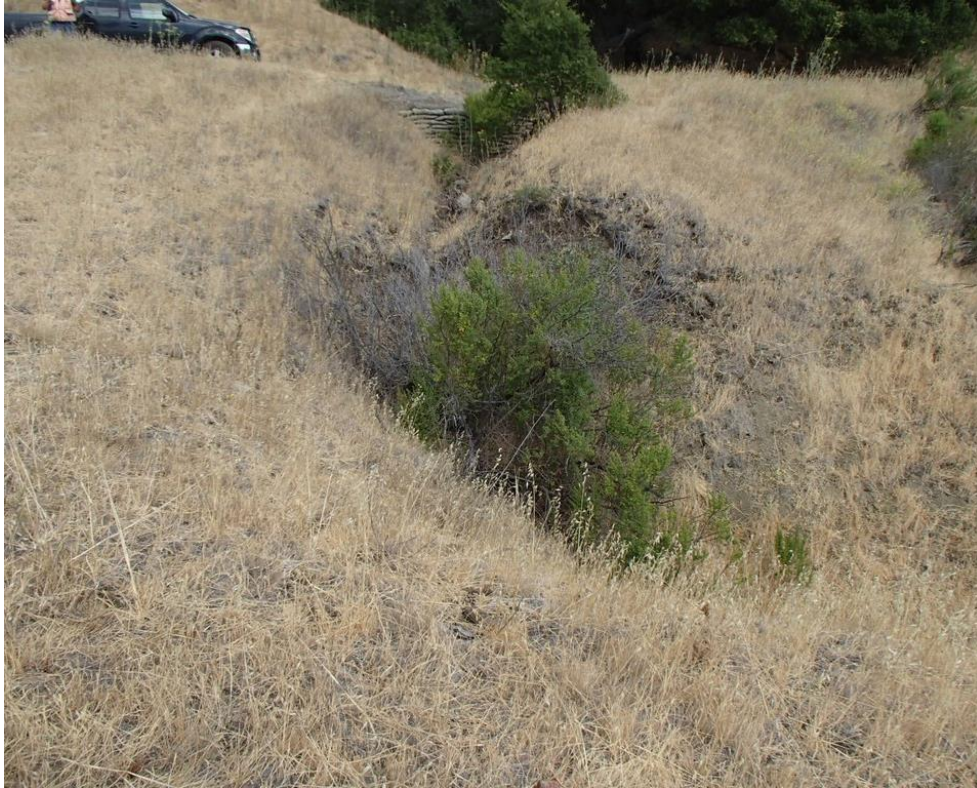
Photo 13. Site 196 (Barn Rd.): View of Site 196 looking upstream. The outboard fill of this ford crossing is buttressed with solidified sacks of concrete. An erosional gully has formed below the outboard edge.
