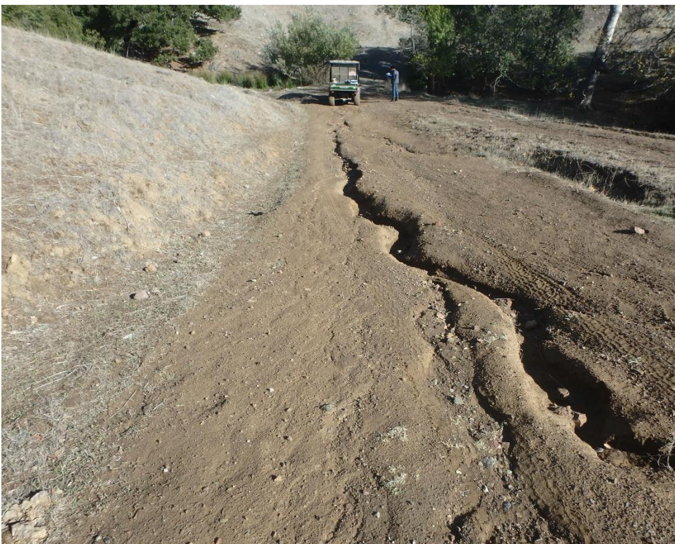
Photo 42. Site 208 (Peterson Ranch Rd.): View of Site 208 road approach looking down the right road approach with stream crossing located in the upper frame. Two gullies have formed on the road surface from excessive road drainage, which funnel sediment to the stream.
