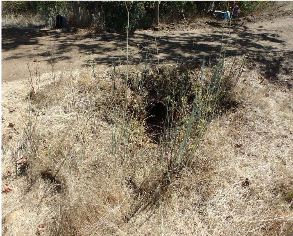
Photo 75. Site 224 (Peterson Ranch Rd.): View of Site 224 looking downstream at the culvert inlet. This culvert is undersized and visible in the center of the frame.
