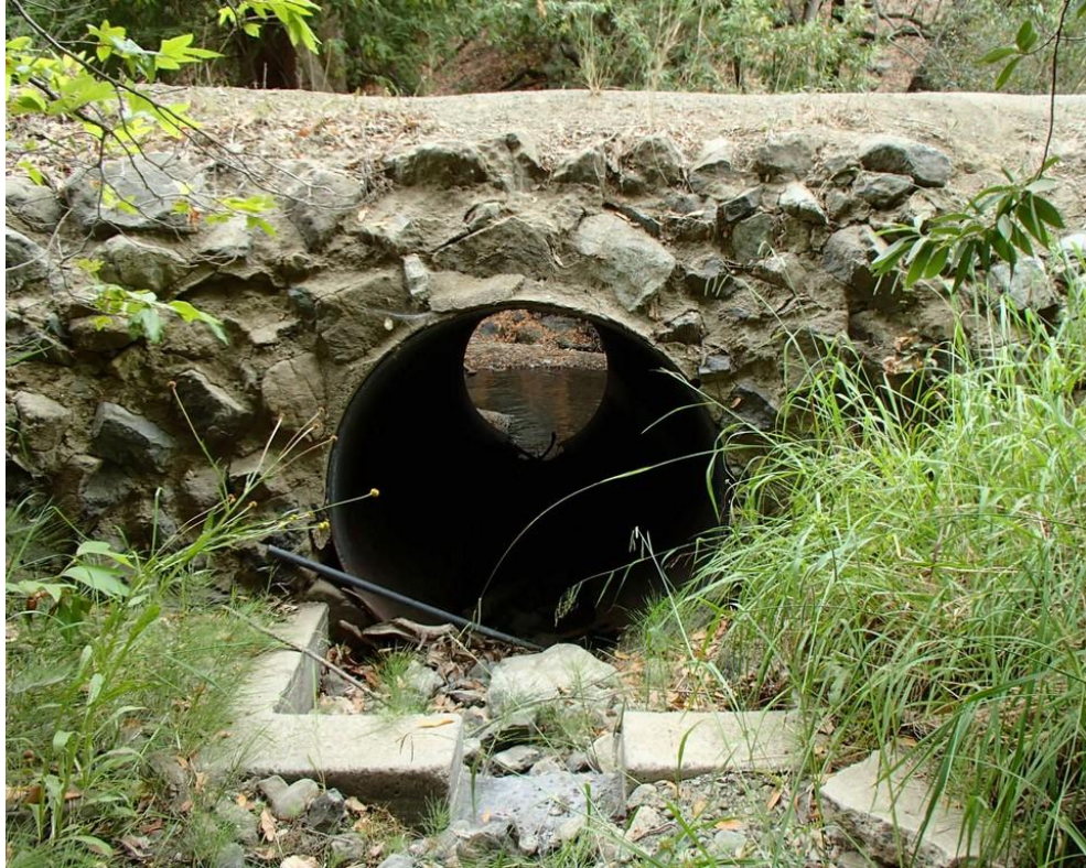
Photo 89. Site 230 (Poly Canyon Rd.): View of Site 230 culvert inlet and road crossing. Looking downstream at mainstem Brizziolari Creek. This culvert is not aligned properly with the stream channel.
