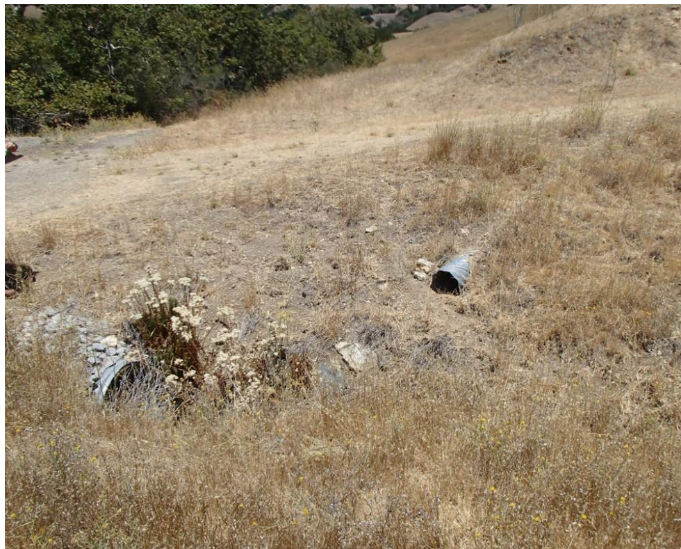
Photo 22. Site 198.1 (Barn Rd.): View of Site 198.1 looking obliquely/upslope at the ditch relief culvert outlet. The culvert outlet is visible in the middle of the frame and the road is above. Site 199 culvert inlet is located on the left.
