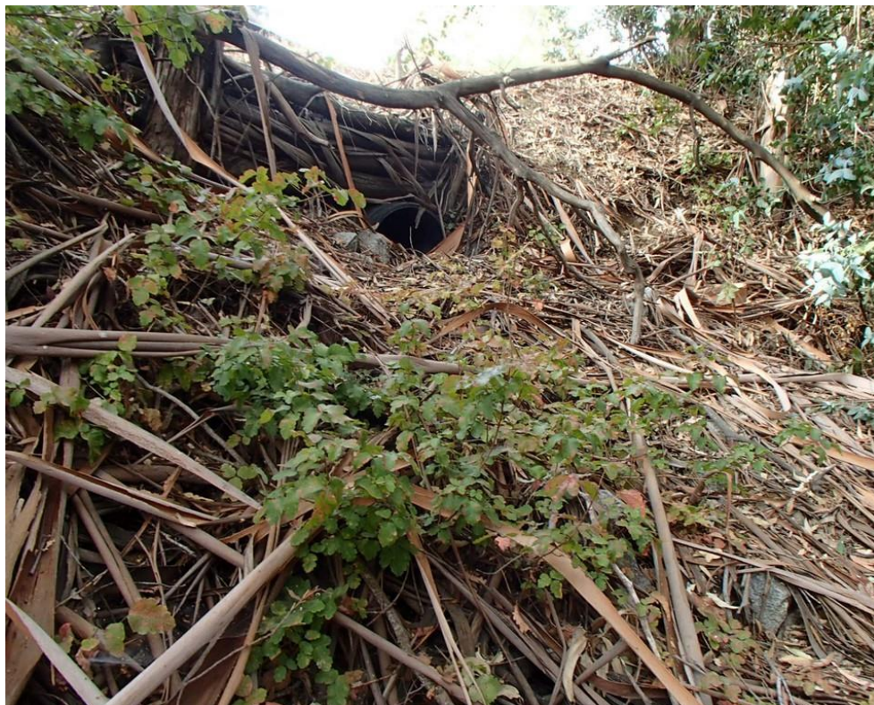
Photo 94. Site 232 (Poly Canyon Rd.): View of site 232 ditch relief culvert outlet area. Looking upslope, the culvert outlet is protruding from a crib wall built of eucalyptus branches at the top-center of the frame.
