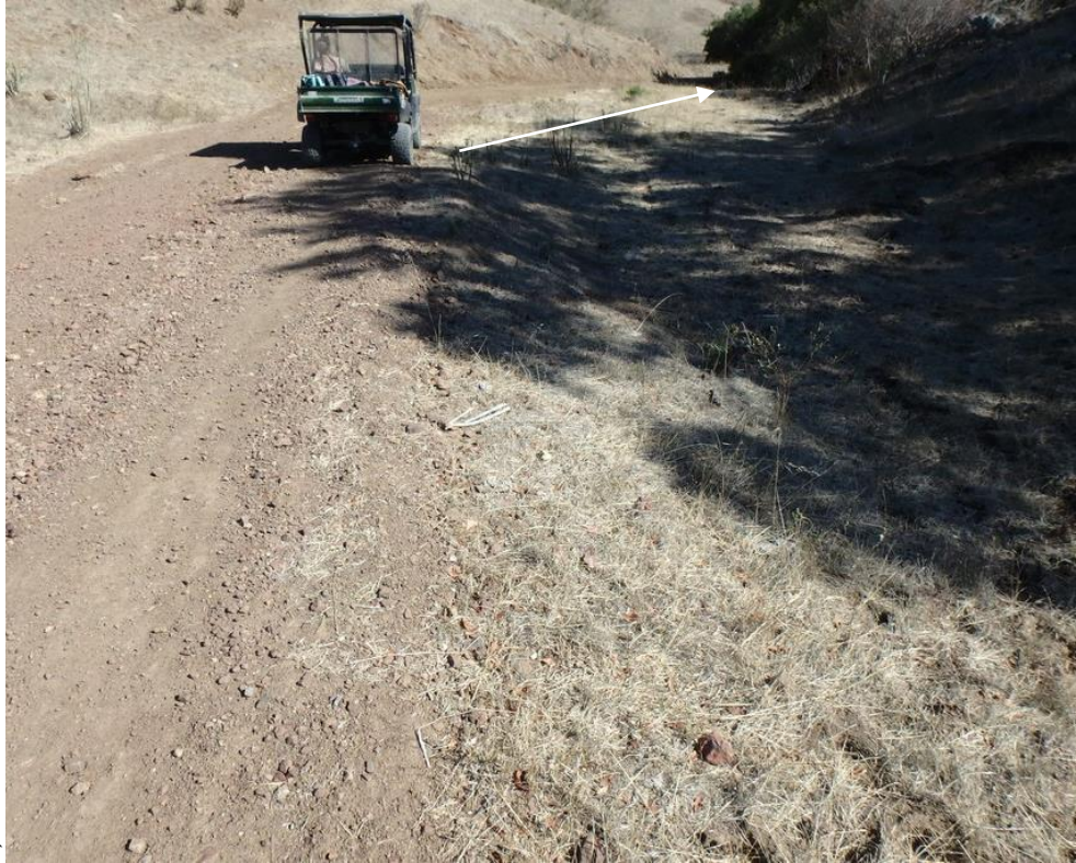
Photo 55. Site 215 (Peterson Ranch Rd.): View of Site 215 looking towards the discharge point and the headwaters area of a Class III stream (see arrow). Concentrated road and hillslope runoff exits the road at this location.
