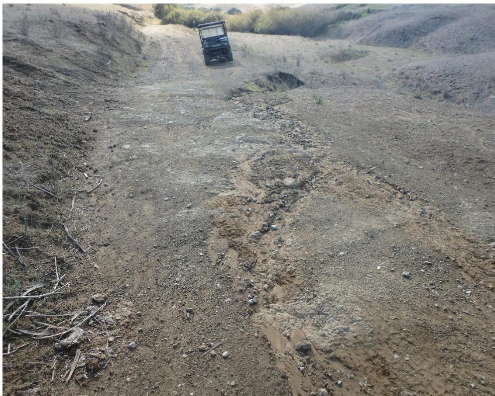
Photo 40. Site 207 (Peterson Ranch Rd.): View of Site 207 looking down the right road towards the road surface discharge point and subsequent gully. Note that fine sediment generated from road surface erosion is being transported down road via a gully in the roadbed.
