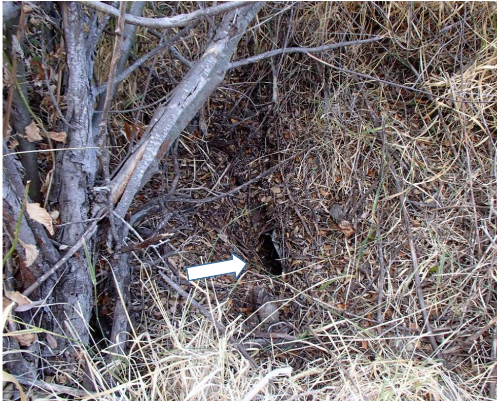
Photo 15. Site 197 (Barn Rd.): View of Site 197 looking obliquely at ditch relief culvert outlet. The culvert outlet is at the center of the frame and is approximately 90% plugged with organic matter (see arrow). The stream flows from right to left.
