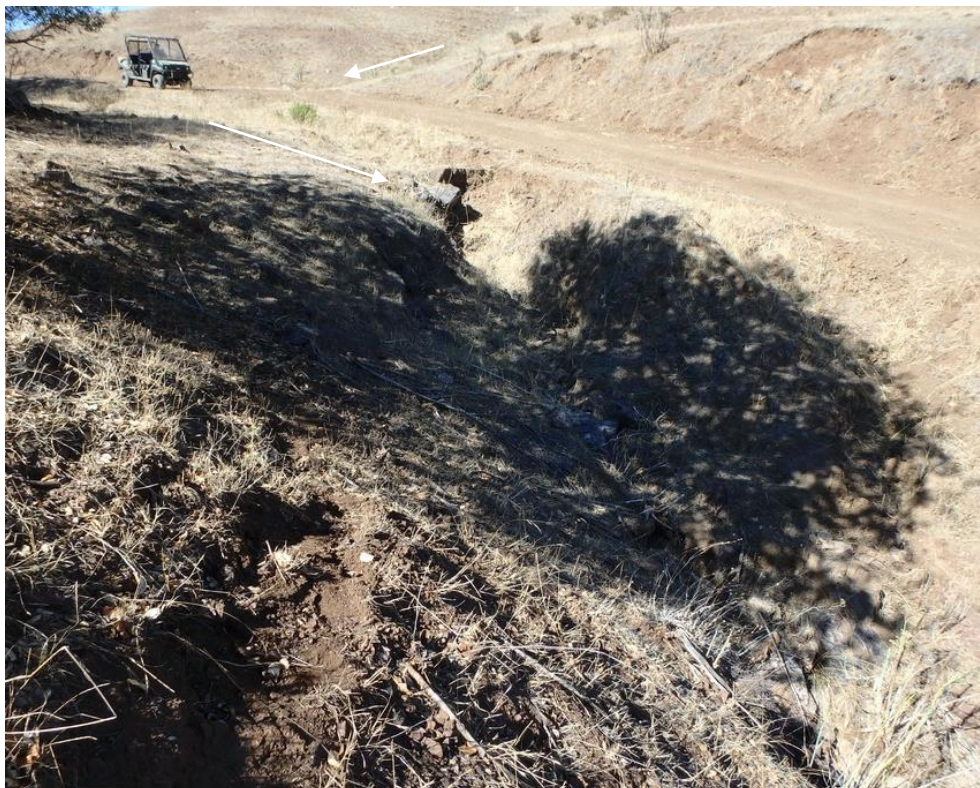
Photo 56. Site 215 (Peterson Ranch Rd.): View of Site 215 looking upslope at the road surface discharge point. The contributing swale is visible in the top of the frame (see arrow).
