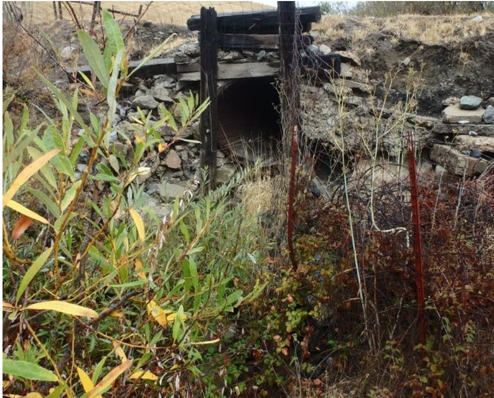
Photo 37. Site 206 (Peterson Ranch Rd.): View of Site 206 looking downstream at the culvert inlet area. The inboard fill area has been shored up by old railroad ties and concrete.
