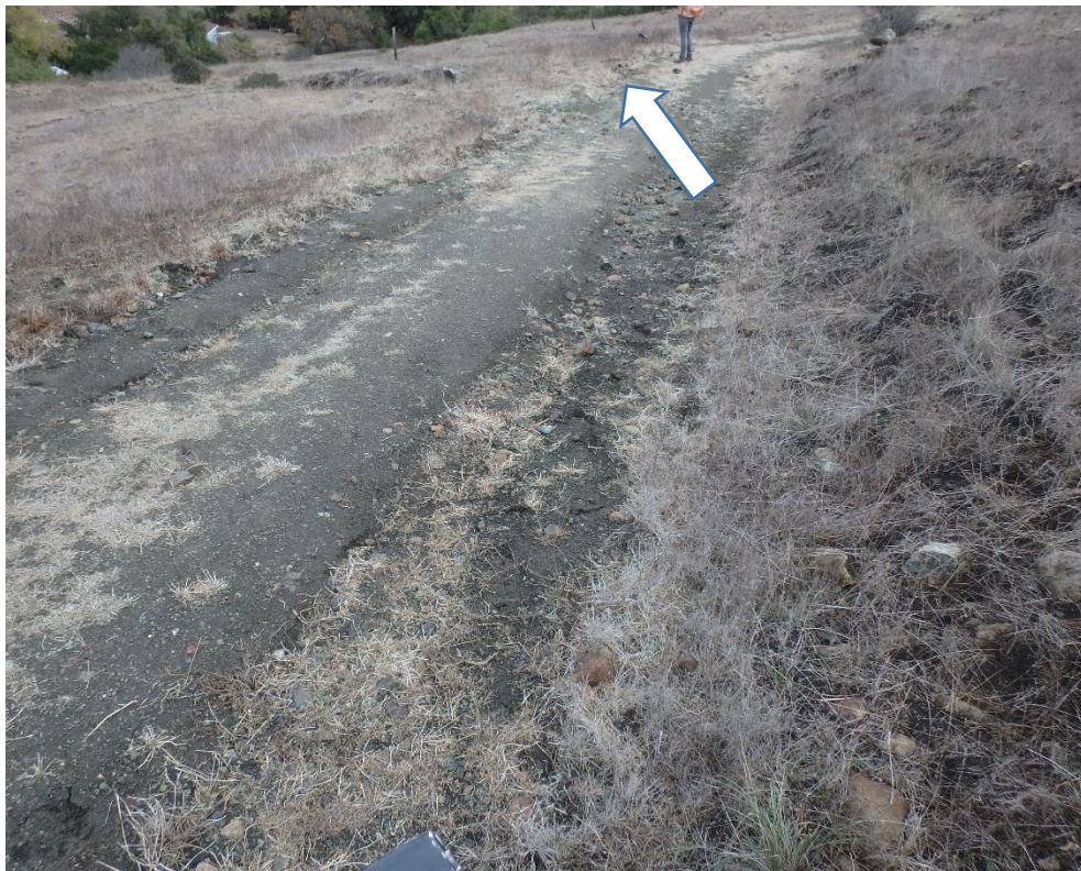
Photo 12. Site 195.3 (Powerline Rd.): View of Site 195.3 looking down the left road towards the road surface discharge point. The discharge point and subsequent gully are visible in the upper left corner of the frame (see arrow).
