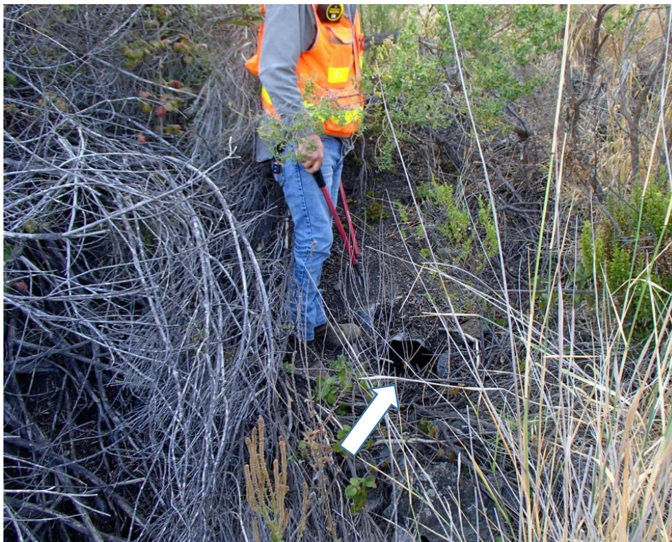
Photo 16. Site 197 (Barn Rd.): View of Site 197 standing upslope of the ditch relief culvert inlet area. The culvert inlet is visible to the right of the worker's feet and is approximately 25% plugged (see arrow).
