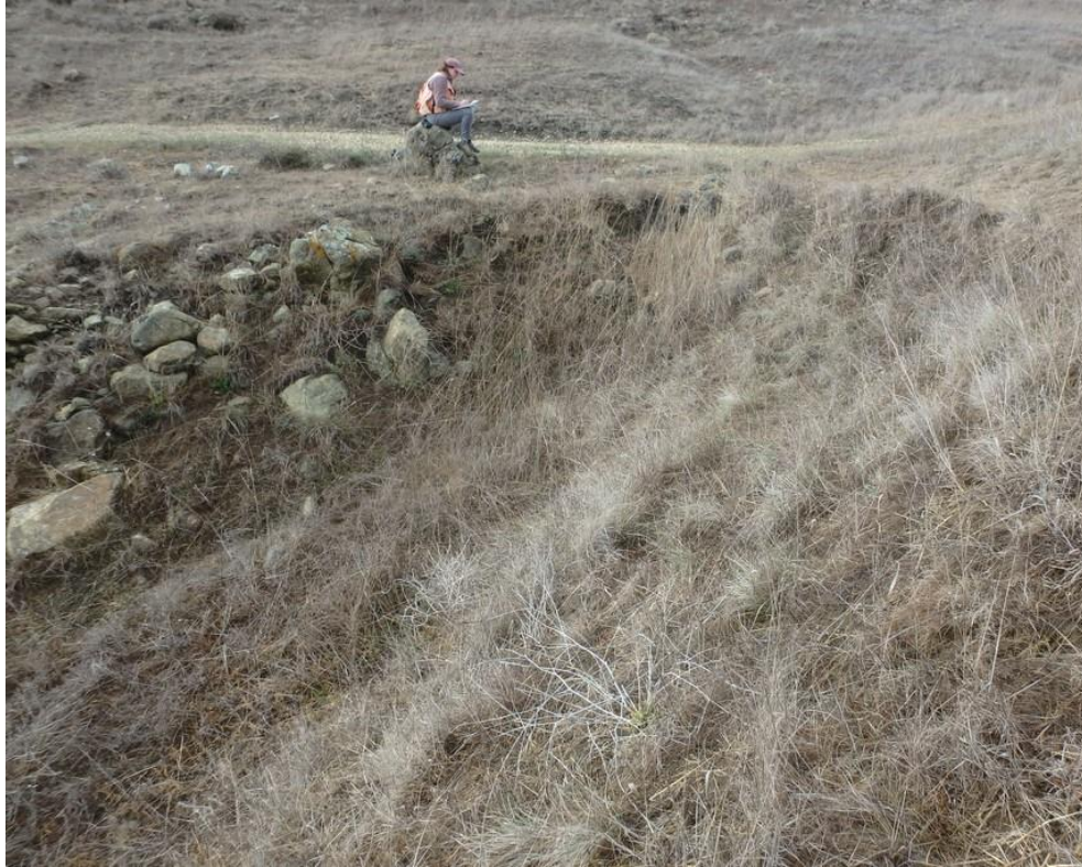
Photo 7. Site 195.1 (Powerline Rd.): View of Site 195.1 looking upstream at the armored fill crossing. Visible in the center of the frame is a headcut that is migrating up towards the outboard road edge.
