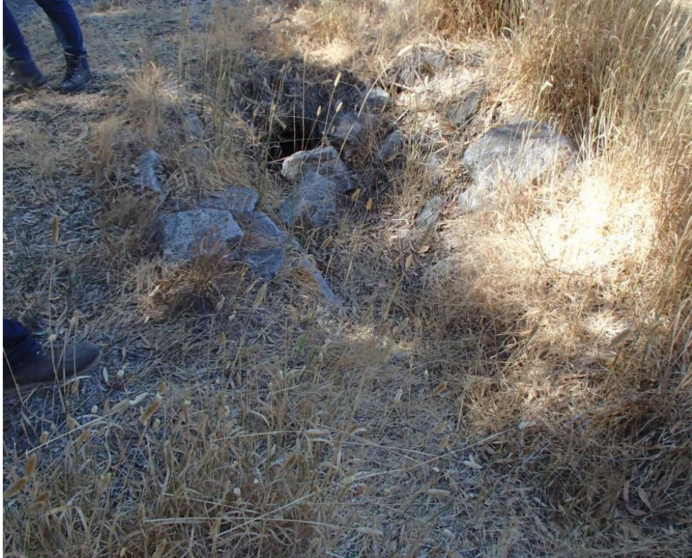
Photo 25. Site 200 (Barn Rd.): View of Site 200 ditch relief culvert inlet area. This culvert inlet is approximately 30% plugged due to the long, wide, and grassy swale that feeds this location.
