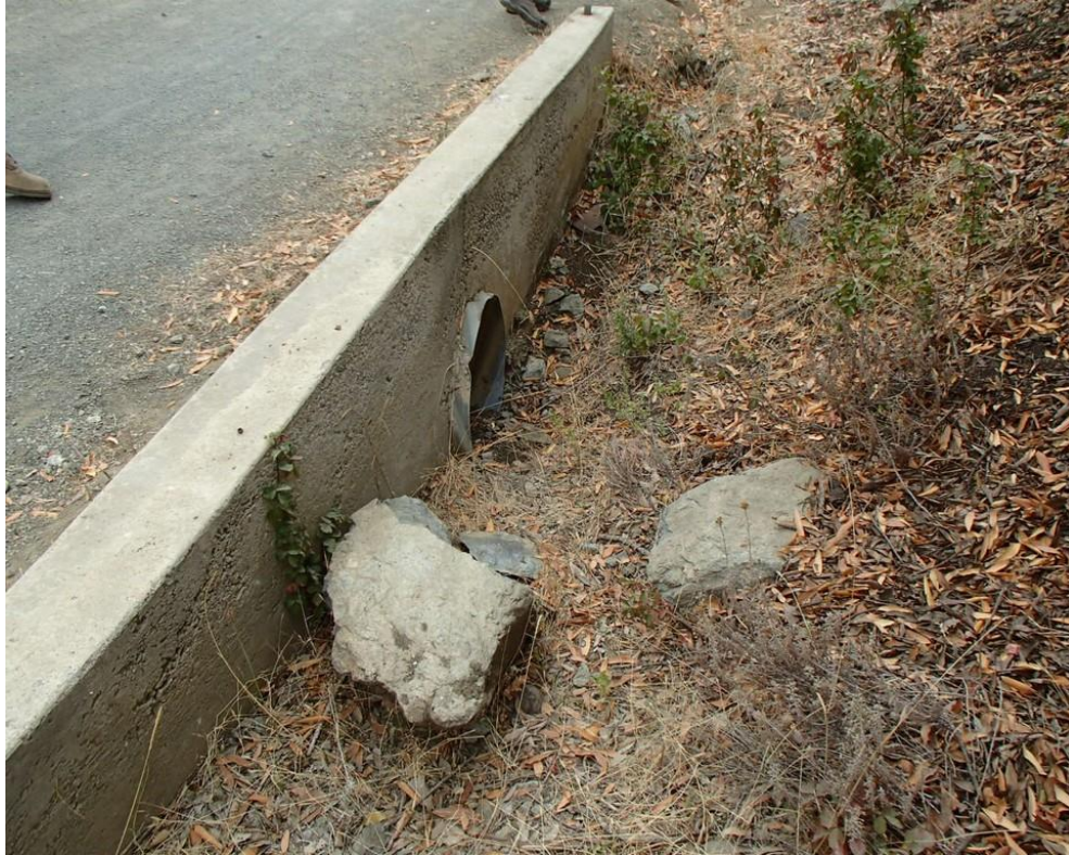
Photo 93. Site 231 (Poly Canyon Rd.): View of Site 231 ditch relief culvert inlet area. The inlet of the culvert has been embedded in a short concrete wall. Site 230.1 diverts to this location along the right road (upper frame).
