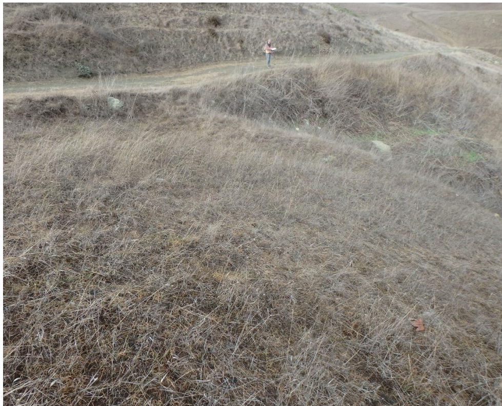
Photo 10. Site 195.2 (Powerline Rd.): View of Site 195.2 looking at the outboard edge of the fillslope. This area has erodible soils and is saturated from emergent springs. The steep fillslope should be monitored for potential failure.
