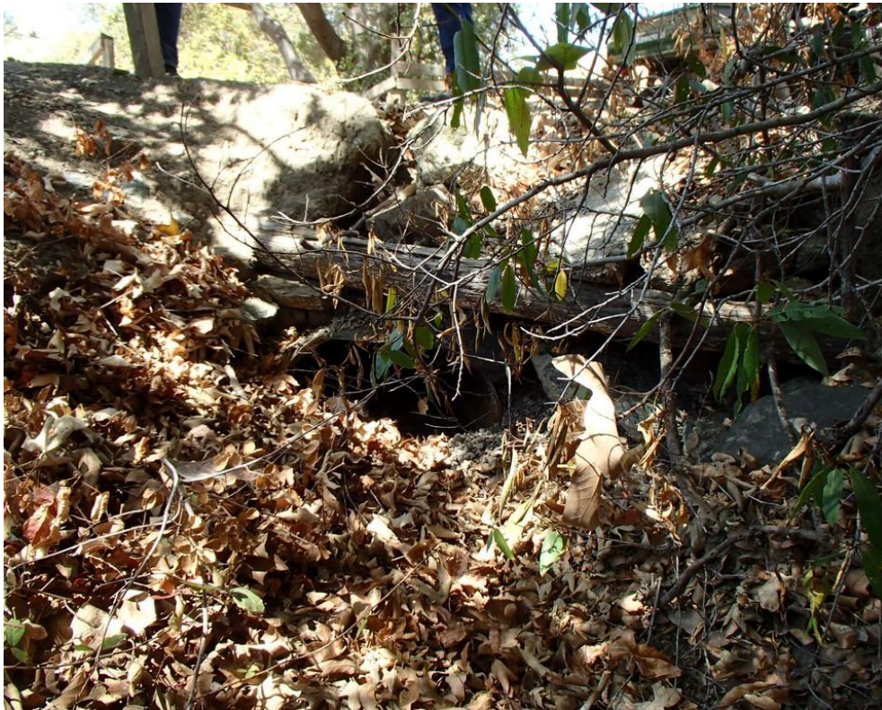
Photo 2. Site 193 (Architectural Canyon Complex Rd.): View of Site 193 looking upstream. The plugged culvert outlet is visible in the center, the road crossing, and road gravel discharge load are in top of the frame.
