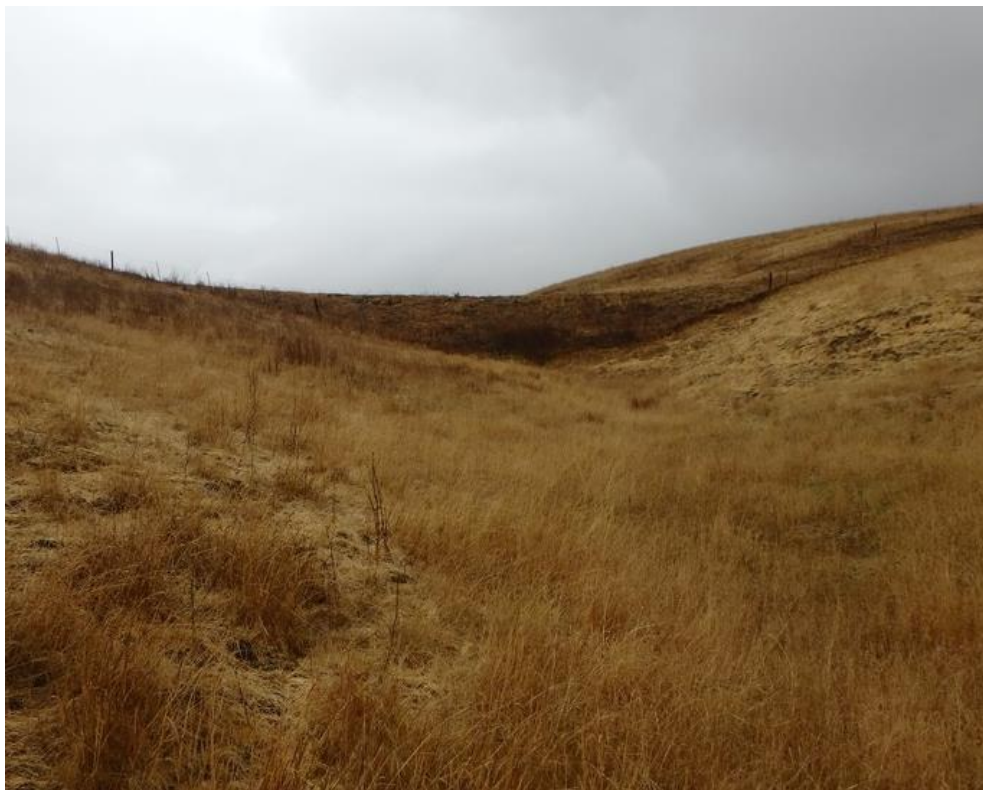
Photo 36. Site 205 (Peterson Ranch Rd.): View of Site 205 looking upstream. The culvert outlet is plugged with silt and is overgrown with vegetation. The outboard edge of the road fill is visible in center of the frame.
