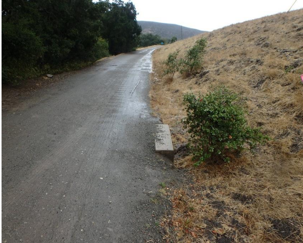
Photo 103. Site 237 (Stenner Creek Rd.): View of Site 237 looking down the right road. Muddy water is visibly ponding and draining into the inlet with concrete headwall in the center of the frame. Mainstem Stenner Creek is located to the left and runs parallel to the road.
