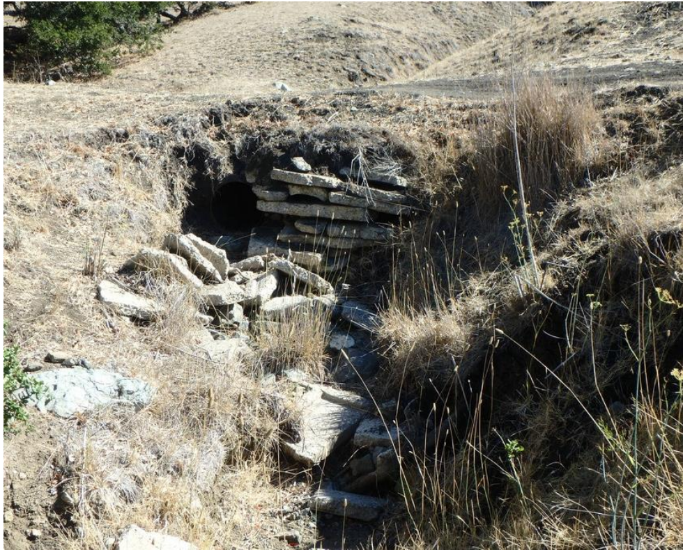
Photo 45. Site 210 (Peterson Ranch Rd.): View of Site 210 looking upstream at the undersized culvert outlet. Concrete blocks and eroding fill are visible in the center of the frame. Upper channel area is visible in the top of frame.
