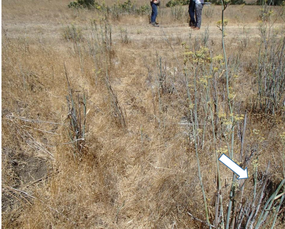
Photo 17. Site 197.1 (Barn Rd.): View of Site 197.1 looking downstream. The culvert inlet is plugged in this location and not easily discernible (see arrow). The road crossing is visible in the top of the frame.
