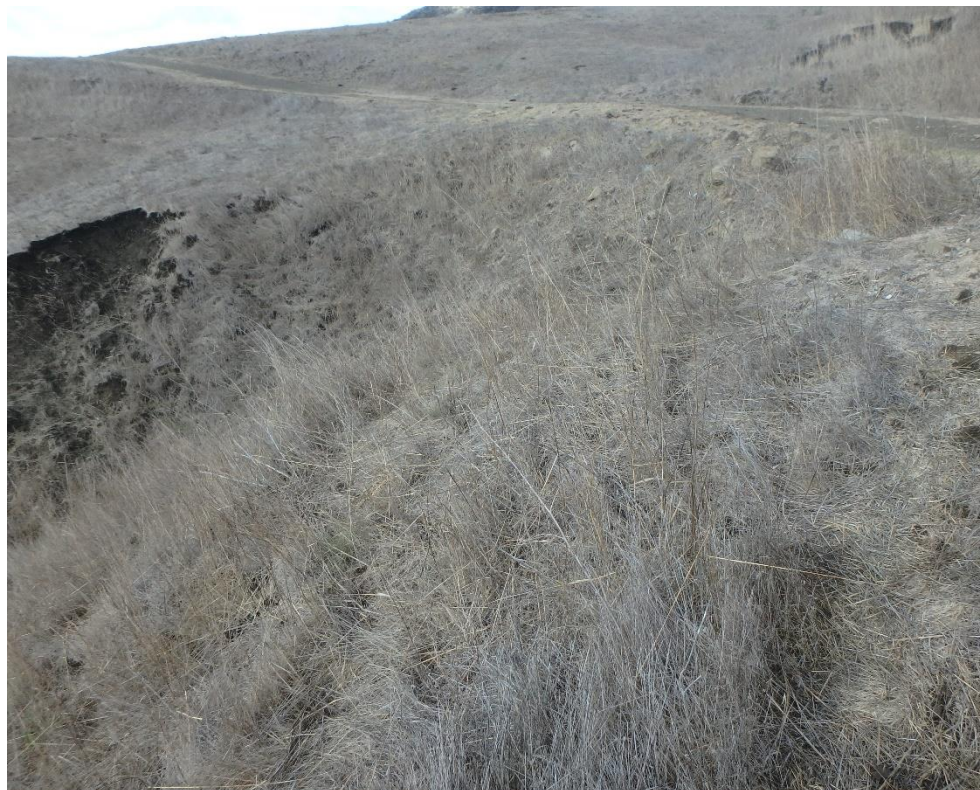
Photo 80. Site 226 (Peterson Loop Spur): View of Site 226 looking up the right road and outboard fill edge. The failing fill edge is visible in the upper half of the frame.
