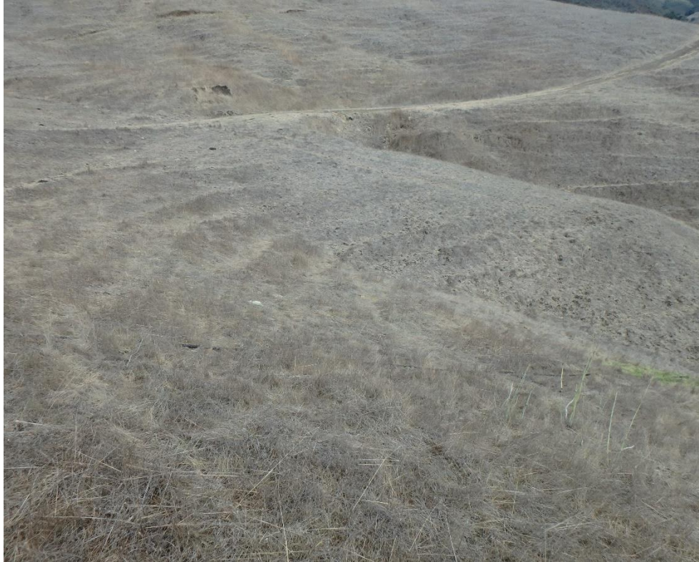
Photo 79. Site 226 (Peterson loop Spur) View of Site 226 looking towards outboard edge of fill. The fill in this location is failing and collapsing into the headwall of the succeeding swale.
