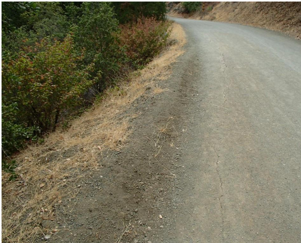
Photo 96. Site 232.1 (Poly Canyon Rd.): View of Site 232.1 looking northeast at tension cracks in road.
