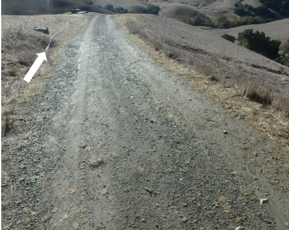
Photo 77. Site 225 (Peterson Ranch Rd.): View of Site 225 looking down road towards mainstem Brizziolari Creek. A plugged ditch relief culvert inlet is visible in the upper lefthand side of the frame (see arrow).
