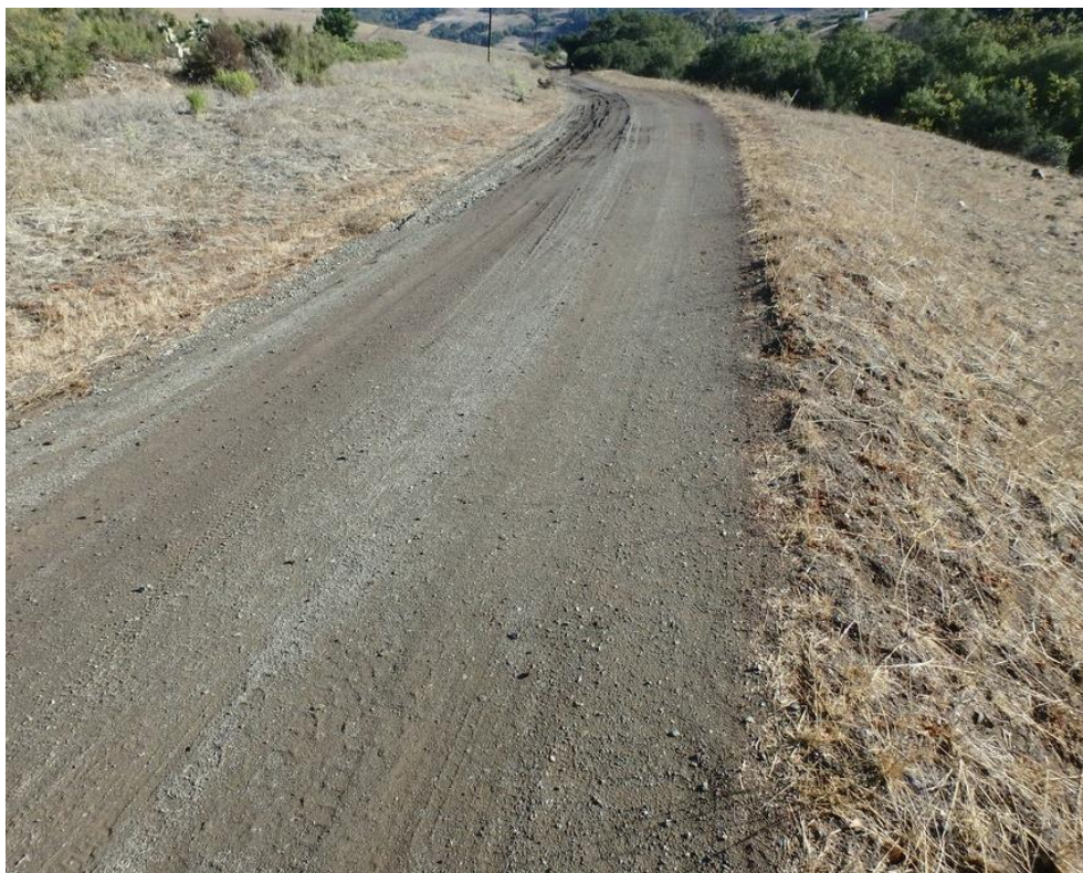
Photo 108. Site 238.1 (Stenner Creek Rd.): View of Site 238.1 road approach, looking up road. The insloped road concentrates road and hillslope runoff to a stream crossing located just outside of Cal Poly property.
