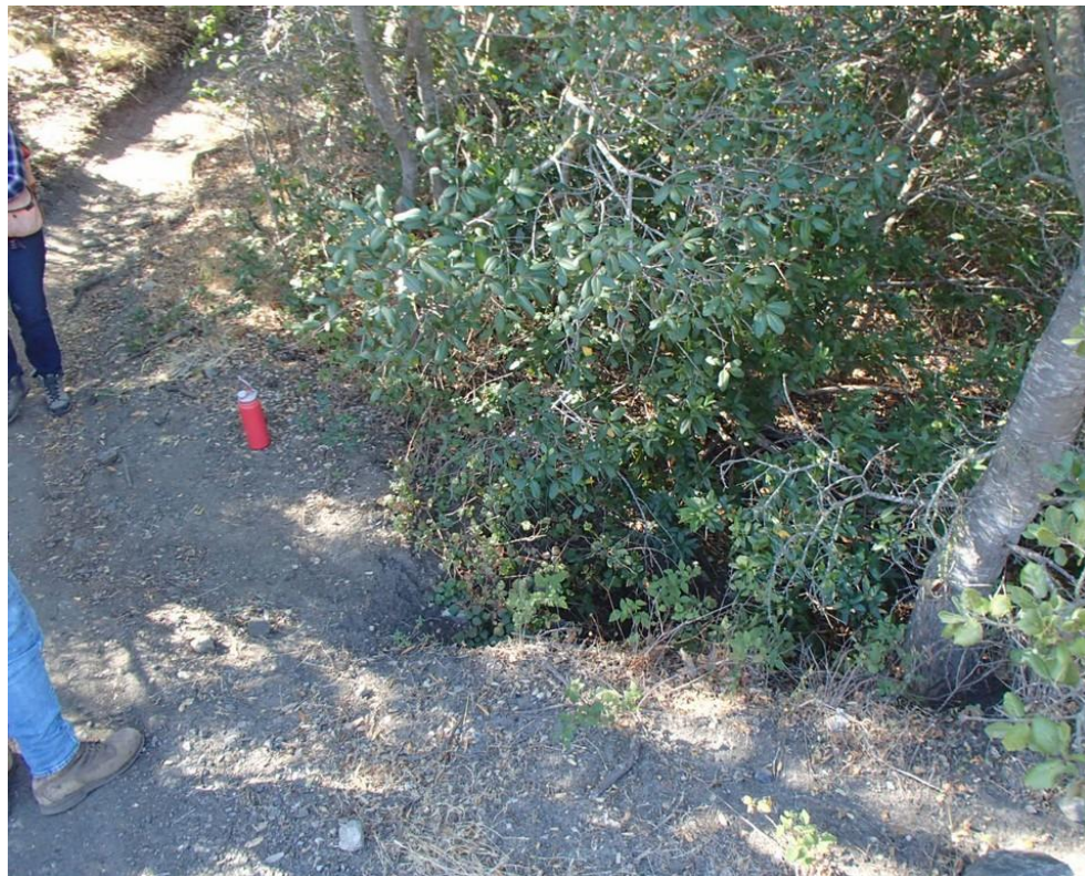
Photo 110. Site 410 (Yewks Trail): View of Site 410 stream crossing looking obliquely at the stream crossing. The downstream gully can be seen in this photo migrating into the outboard edge of the trail.
