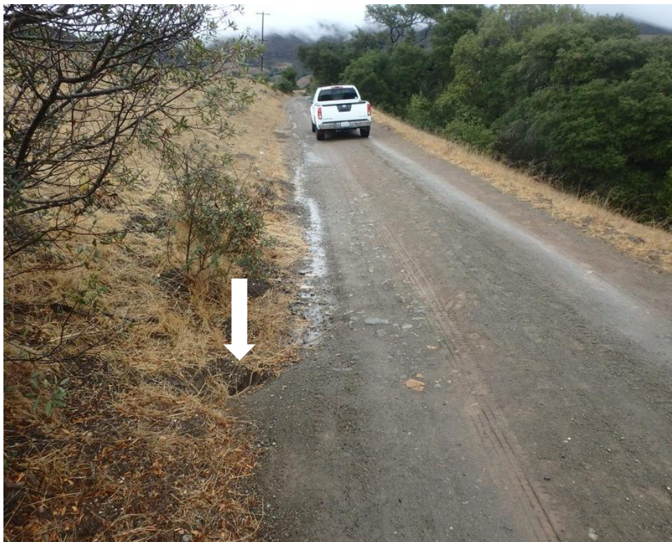
Photo 106. Site 238 (Stenner Creek Rd.): View of Site 238 looking at the ditch relief culvert inlet (see arrow). Muddy water is visibly running down the road and into the culvert. Mainstem Stenner Creek runs parallel to this road on the right side of the frame.
