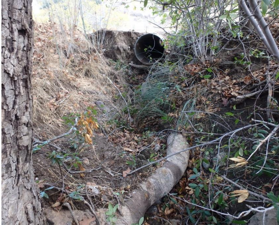
Photo 57. Site 216 (Peterson Ranch Rd.): View of Site 216 looking upstream at the culvert outlet. Erosion is visible on the outboard fillslope and at the base of the culvert due to culvert being installed high in the fill.
