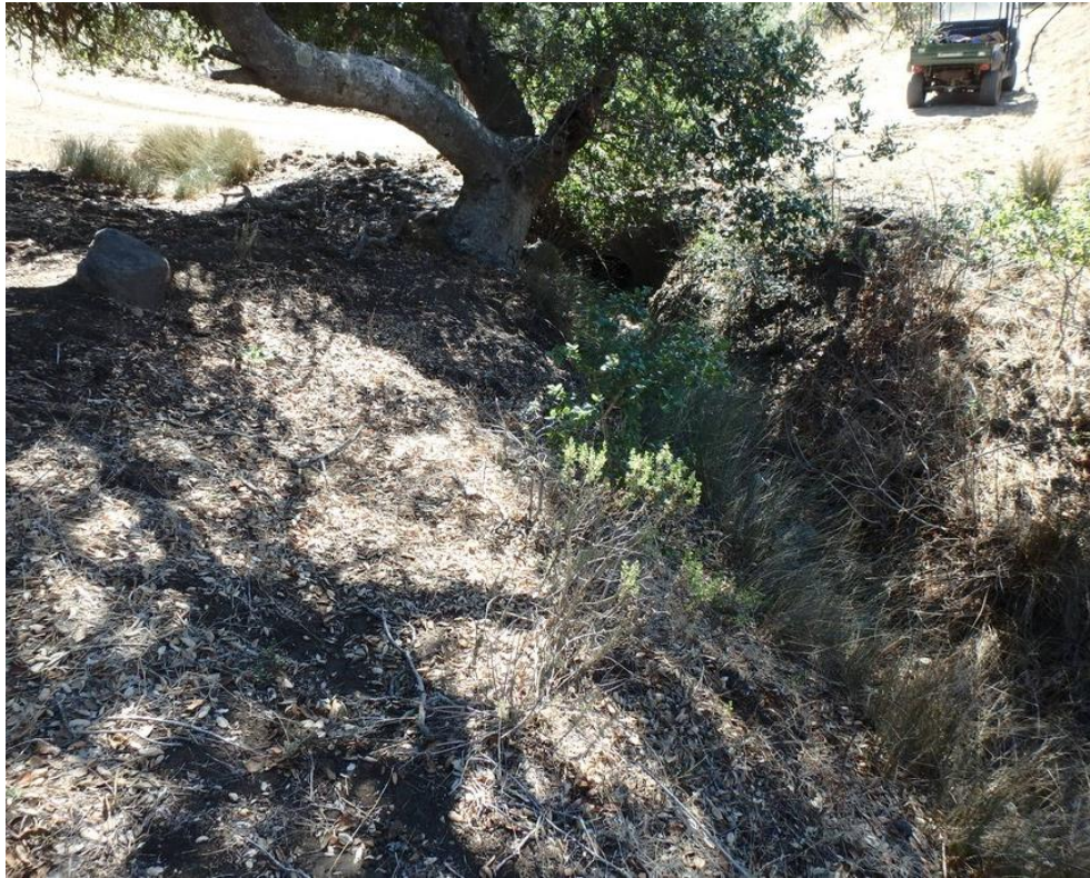
Photo 53. Site 214 (Peterson Ranch Rd.): View of Site 214 looking downstream. The undersized culvert inlet area is visible in the top center of the frame. The Right and left road approaches funnel fine sediment to the site each winter.
