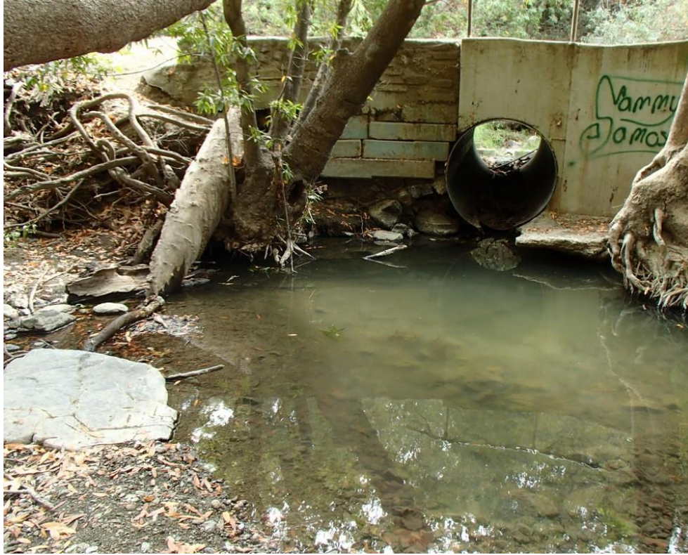
Photo 91. Site 230 (Poly Canyon Rd.): View of Site 230 culvert outlet and road crossing. Looking upstream at mainstem Brizziolari Creek, notice the pool of water at culvert outlet and the erosion on the left side of the frame.
