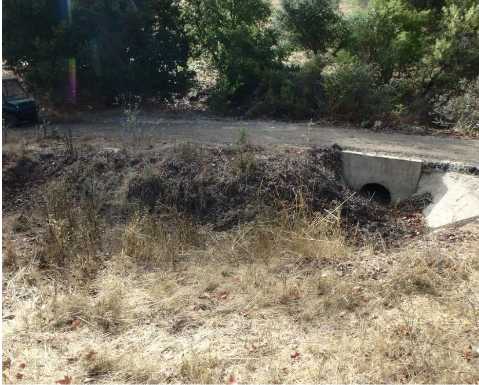
Photo 71. Site 222 (Peterson Ranch Rd.): View of Site 222 looking downstream. Mainstem Brizzolari Creek makes a 90 degree turn at this location, and concrete has been poured on the right bank in an attempt to buttress the slope from erosion.
