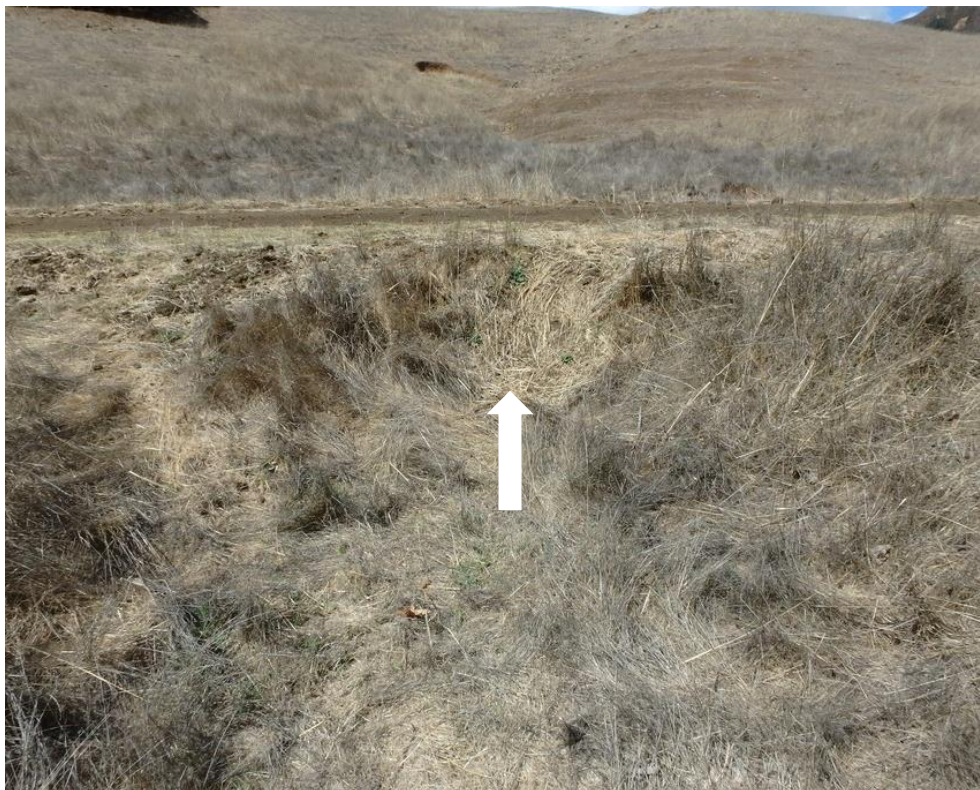
Photo 84. Site 227.1 (Peterson Ranch Rd.): View of Site 227.1 looking at the plugged ditch relief culvert outlet (see outlet). The road crossing is visible at the center of the frame and the swale leading to the culvert is present at the top of the frame.
