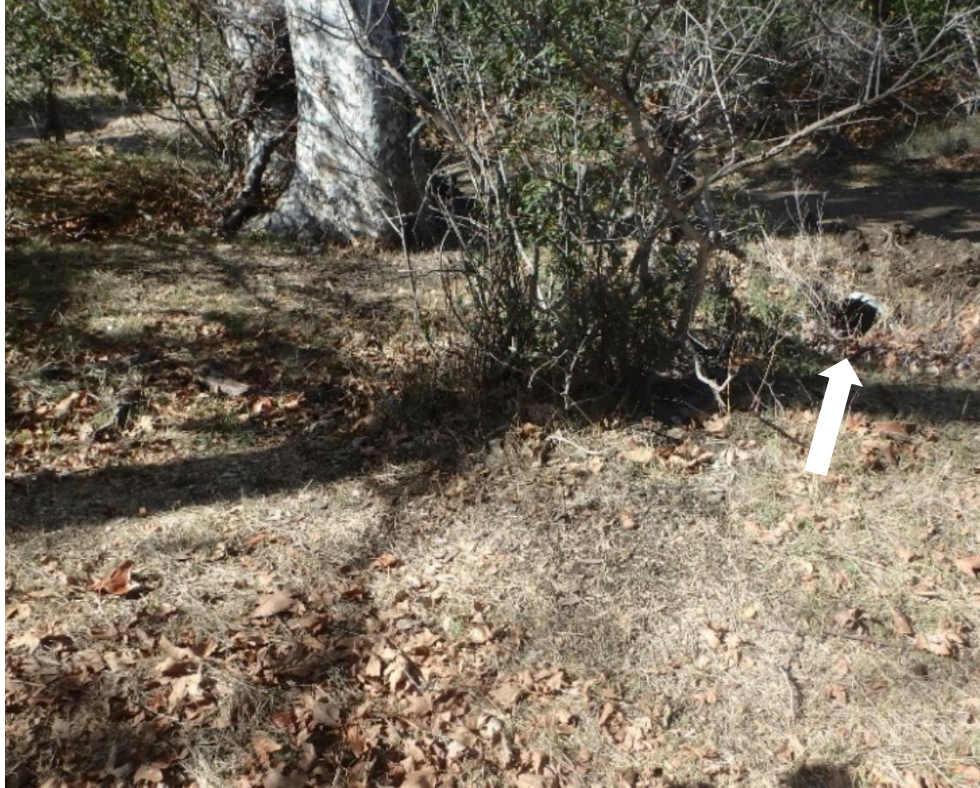
Photo 69. Site 221 (Peterson Ranch Rd.): View of Site 221 looking downstream towards the culvert inlet (see arrow). This undersized culvert is prone to plugging during wet weather events. This culvert discharges directly into Brizziolari Creek.
