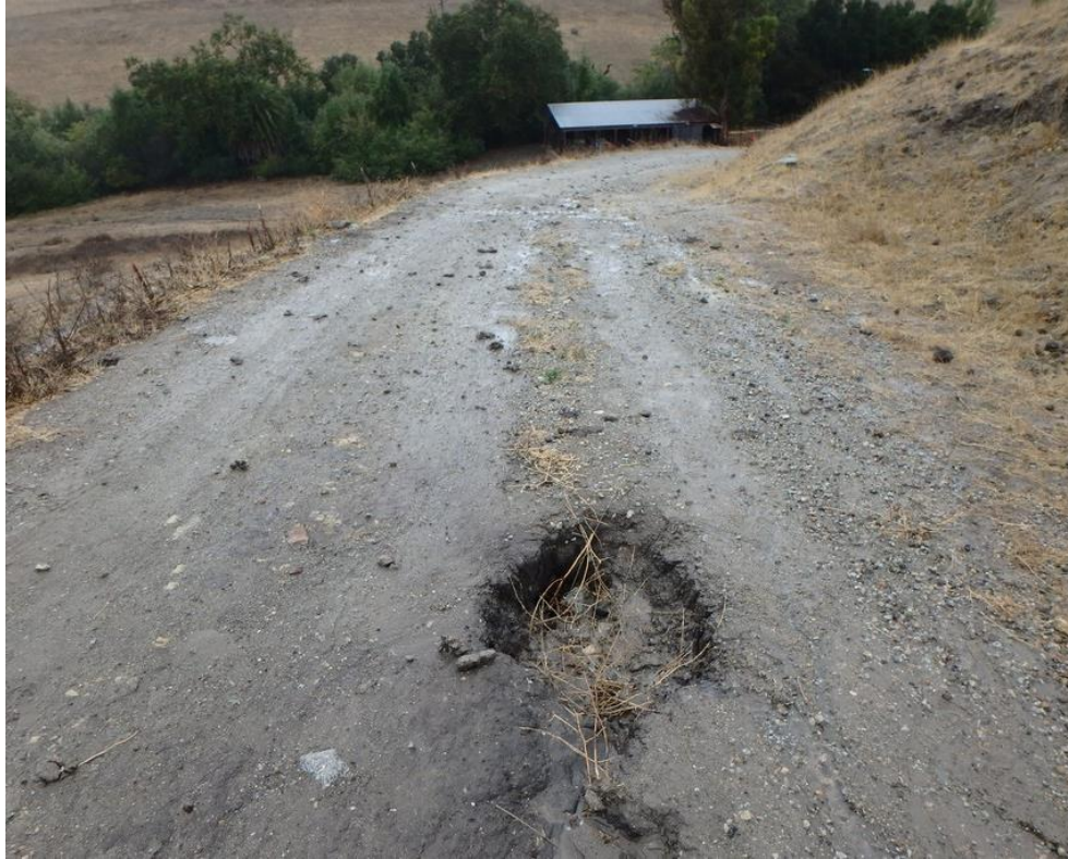
Photo 27. Site 201 (Peterson Ranch Rd.): View of Site 201 looking down left road towards mainstem Stenner Creek. This road approach leads to Site 201 which outlets directly into Stenner Creek. Road erosion is visible in the bottom of the frame.
