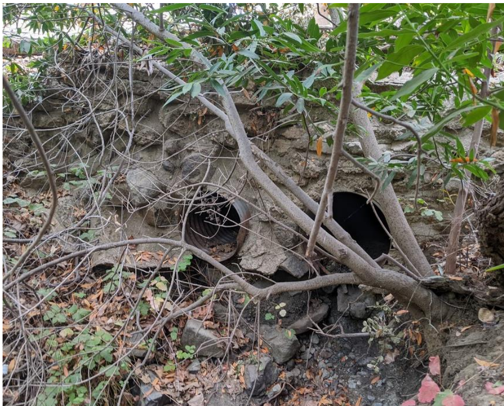
Photo 88. Site 229 (Peterson Ranch Rd.): View of Site 229 culvert outlet area looking upstream. The culverts are not plugged at the outlets but there is evident erosion at the base of the culverts from undercutting.
