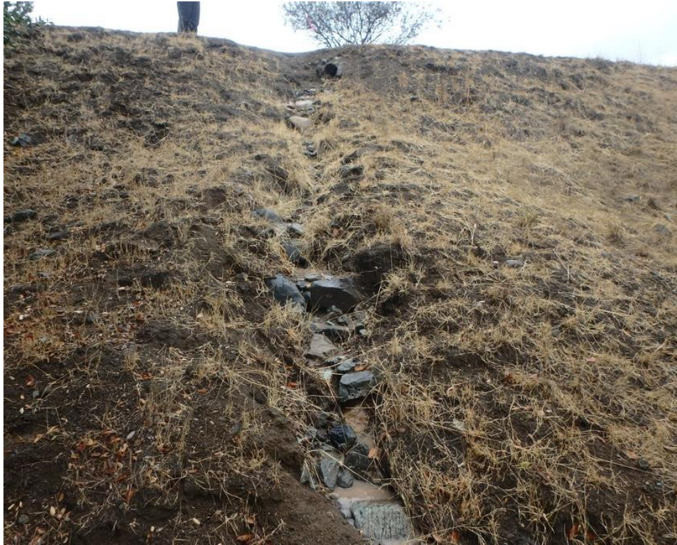
Photo 105. Site 238 (Stenner Creek Rd.): View of Site 238 gully erosion from concentrated road runoff from the ditch relief culvert outlet. Fine sediment and muddy water deliver to mainstem Stenner Creek at this location.
