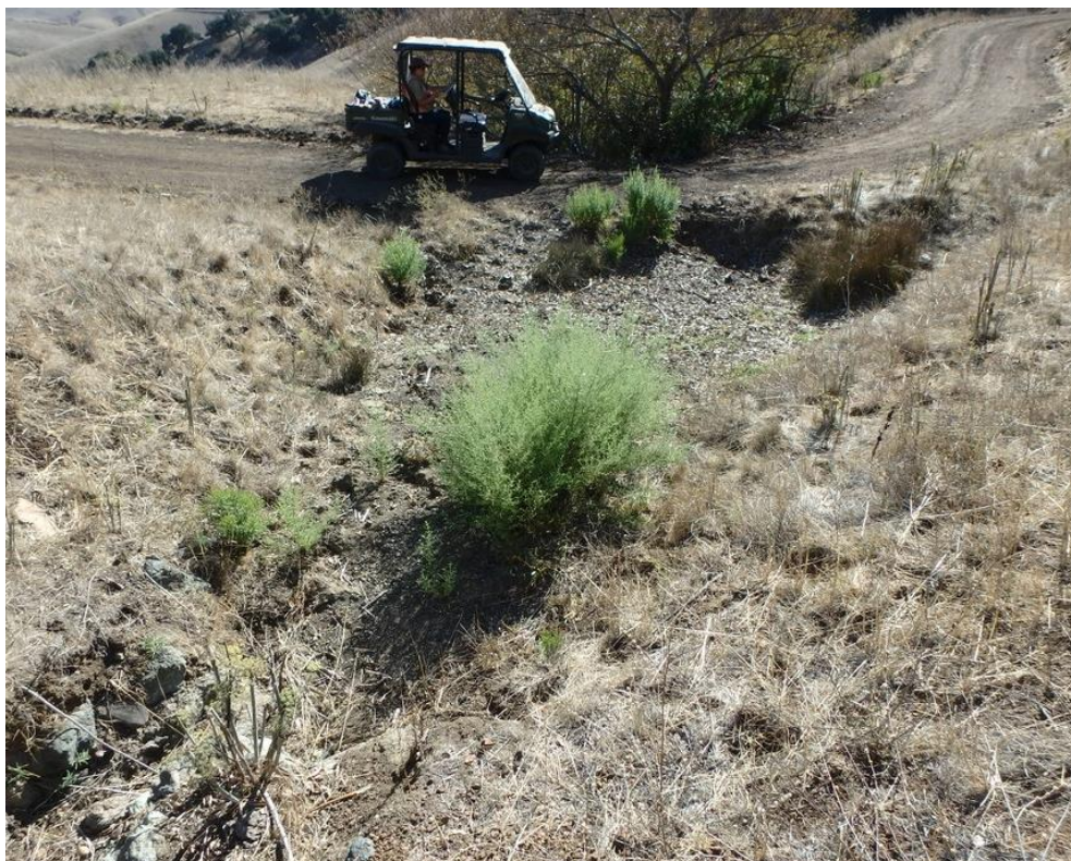
Photo 52. Site 213 (Peterson Ranch Rd.): View of Site 213 looking downstream. The culvert inlet area and aggraded sediment is visible in the middle frame. Both road approaches contribute fine sediment runoff directly to site.
