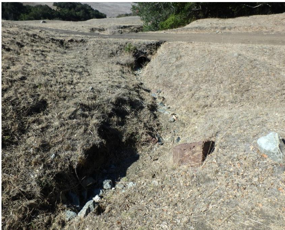
Photo 46. Site 210 (Peterson Ranch Rd.): View of Site 210 looking downstream at the undersized culvert inlet. The stream overtops the road crossing, visible in the top frame, during peak events.
