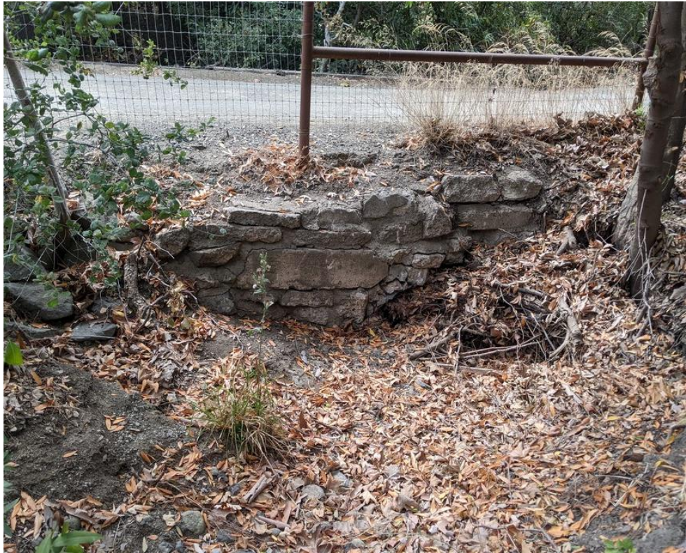
Photo 87. Site 229 (Peterson Ranch Rd.): View of Site 229 looking downstream towards the double culvert inlets that are plugged with detritus. The road crossing is visible at the top of the frame.
