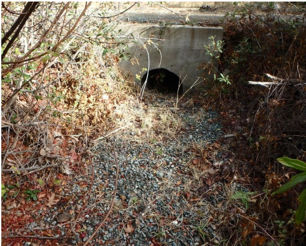
Photo 72. Site 222 (Peterson Ranch Rd.): View of Site 222 looking upstream at the drastically undersized culvert outlet. The road crossing is visible in the top of the frame. Gravel washed into stream can be seen in the center of the frame.
