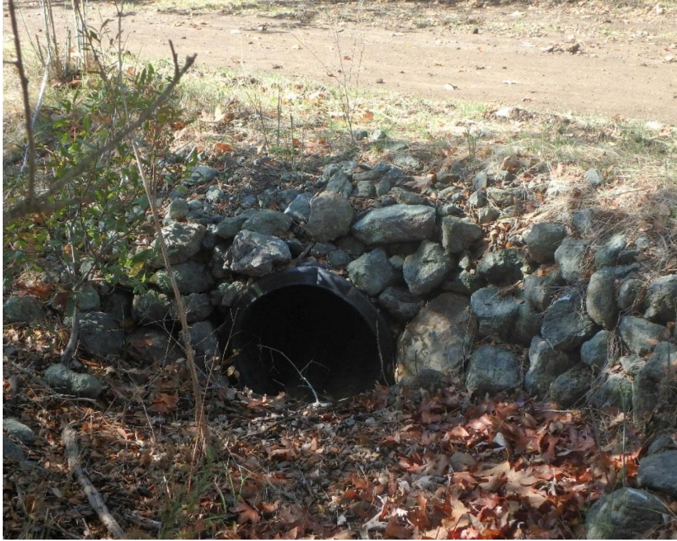
Photo 67. Site 220 (Peterson Ranch Rd.): View of Site 220 looking downstream towards culvert inlet. This undersized culvert is prone to plugging during storm events and discharges directly in Brizziolari Creek.
