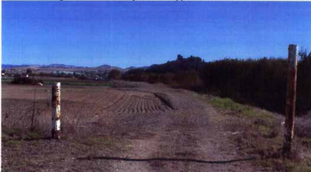
Photo 4: Farmland cutting into north levee top between approximate Stations 103+00 and 103+50 -
