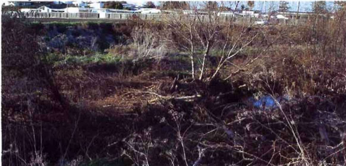
Photo 4: Debris jam from east
