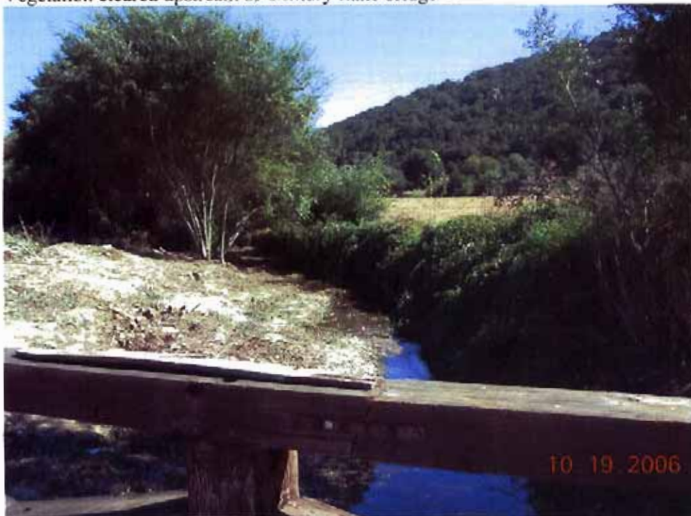
Photo 10: Vegetation cleared upstream of Century Lane bridge –
