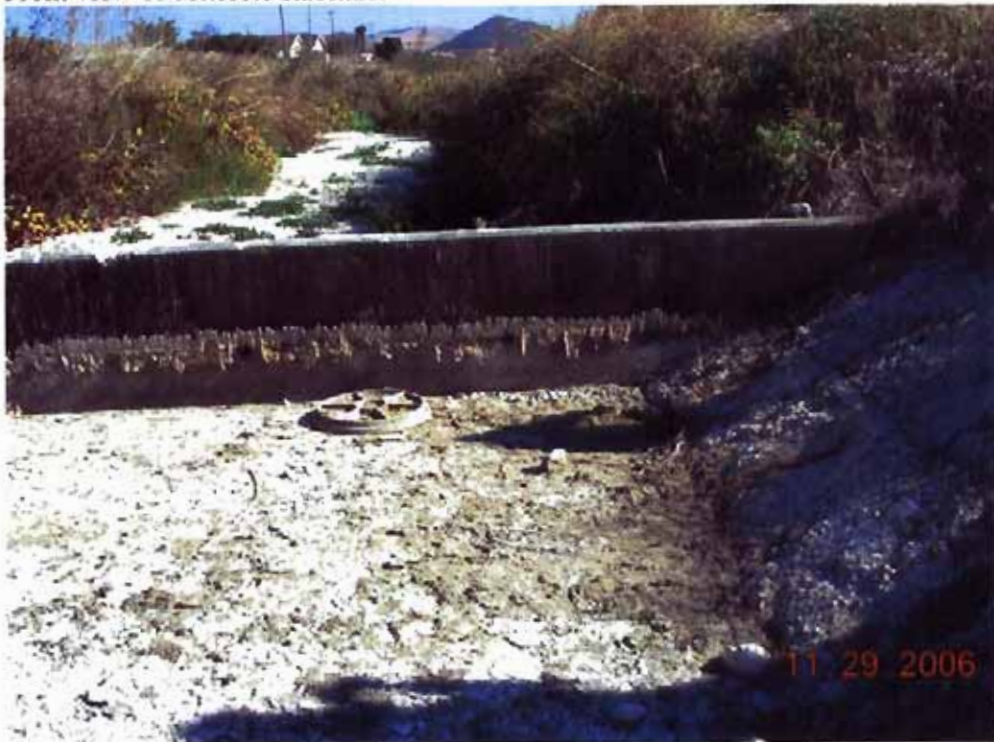
Front view of concrete stabilizer –
