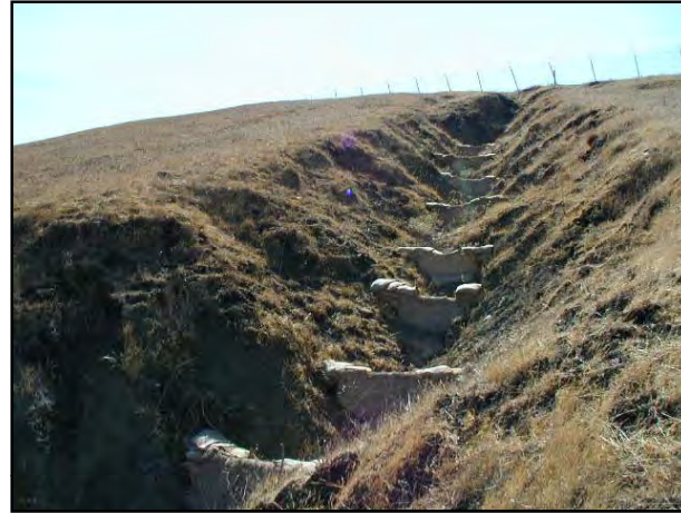
Figure 24. Looking upstream at check dams
