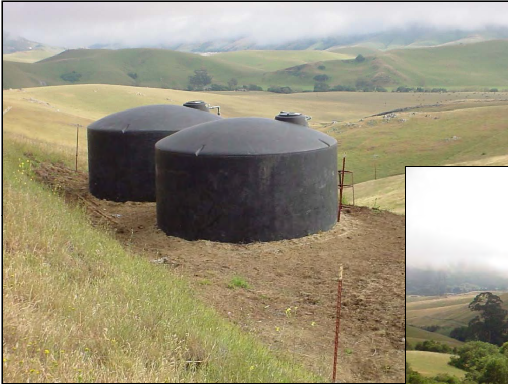
Figure 29. Tanks hold water collected from springs and horizontal well.
