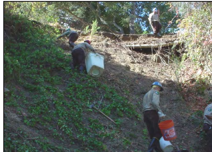
Figure 73. Corps hauling rock & soil out all the way up the hill!
