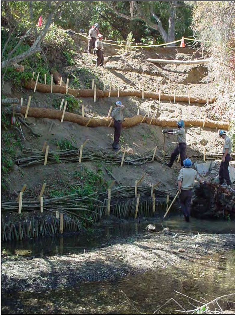
Figure 78. Willow stakes and facines being installed by CCC.
