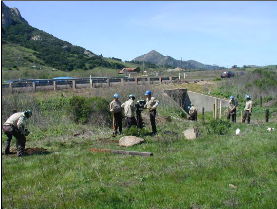
Figure 68. Corps crew installing perimeter fence
