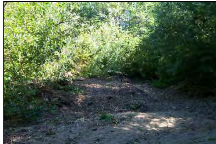
Figure 63. Debris jam in Los Osos Creek after CCC clearing
