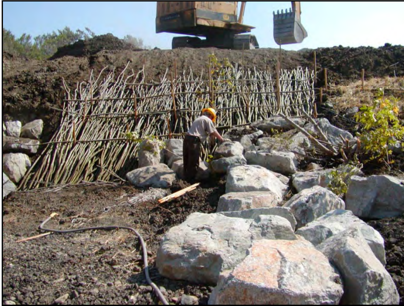
Figure 13. Willow stakes planted along bank.
