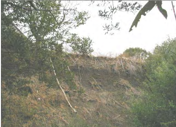
Figure 70. Eroding stream bank.
