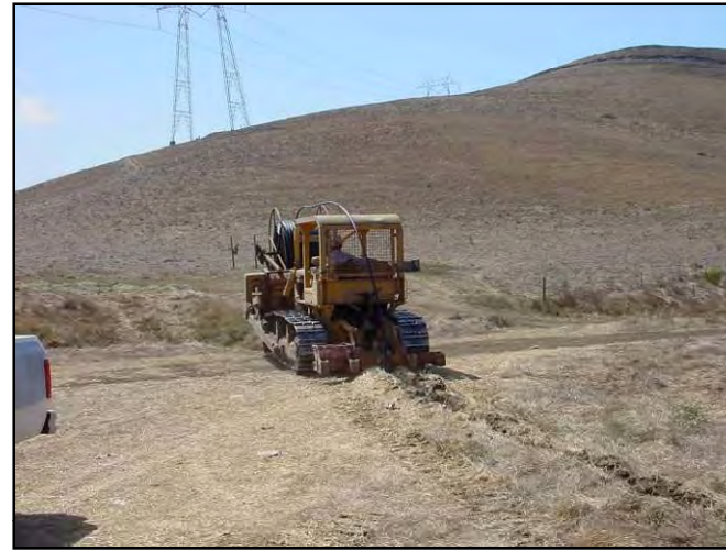
Figure 113. Close-up of cat ripping pipe into ground.
