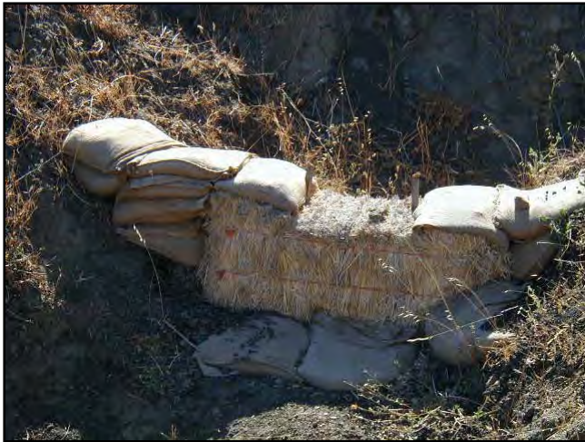
Figure 25. Straw bale and sand bag check dam
