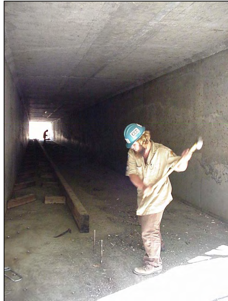
Figure 88. CCC crew member removing baffles.
