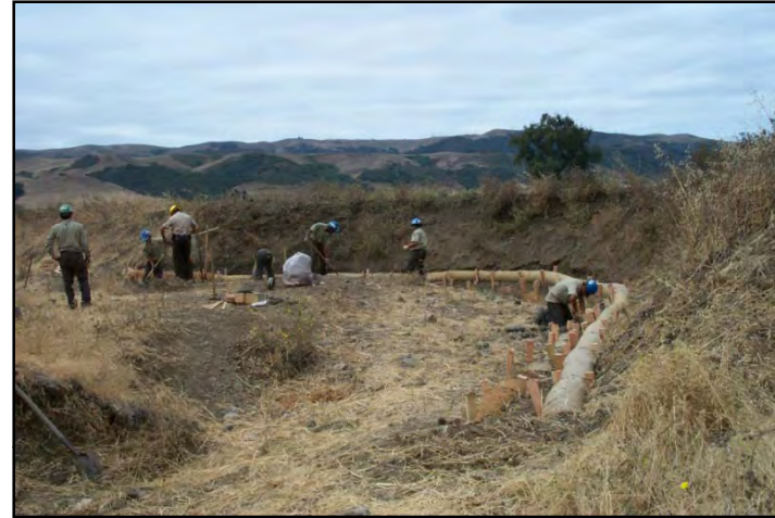
Figure 52. Installing coir logs.
