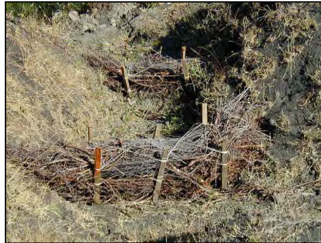
Figure 26. Brush check dam
