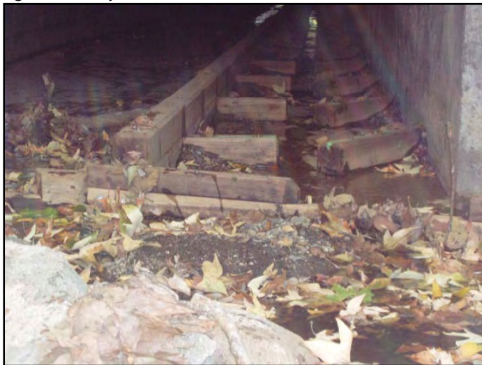
Figure 87. Modified baffles, note they are half as tall as before.
