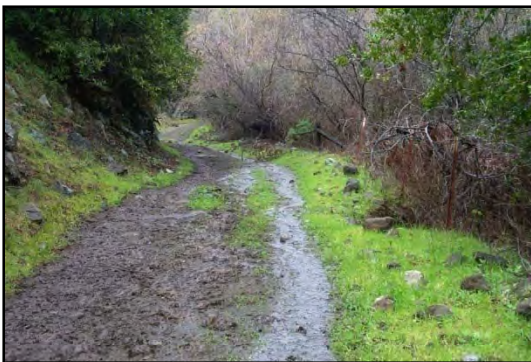
Figure 103. Water running down road.
