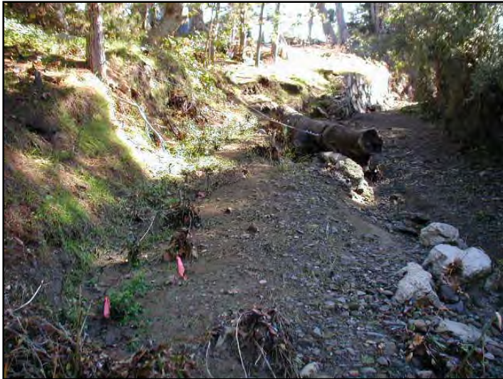
Figure 9. Willow stakes planted along bank.
