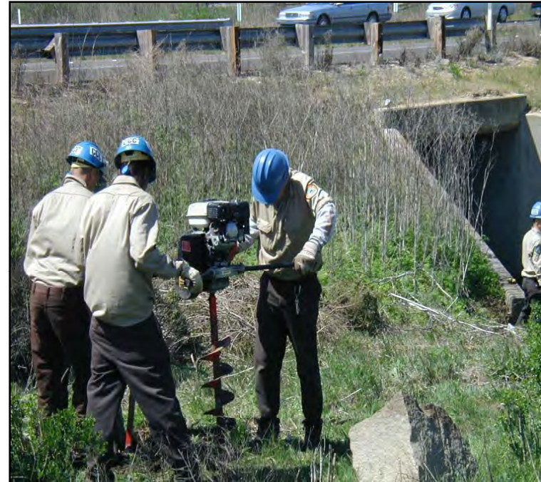
Figure 69. Corps crew installing holes for posts.
