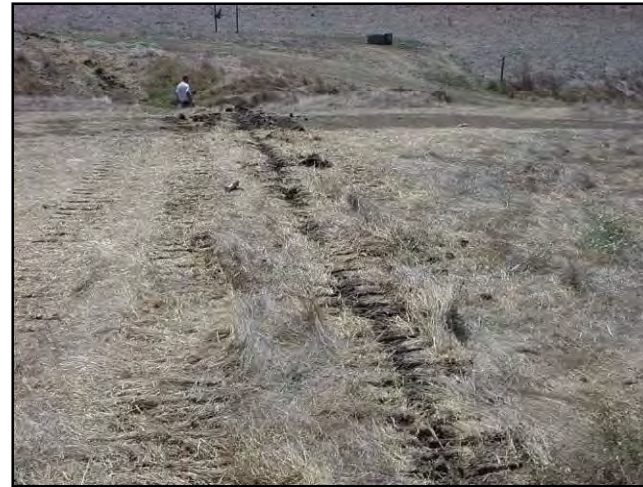
Figure 115. After pipe installation – minimal soil impact.
