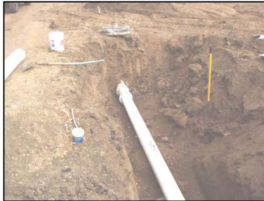
Figure 138. Connected to an existing line.
