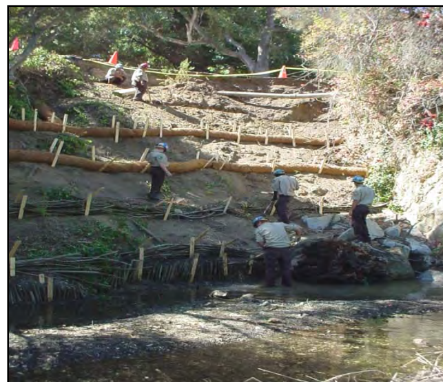
Figure 77. View of bio logs and laid back slope.
