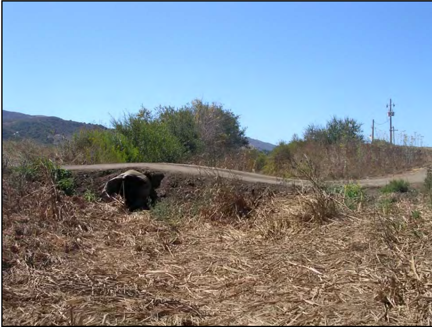
Figure 89. Looking downstream at Warden Creek crossing.
