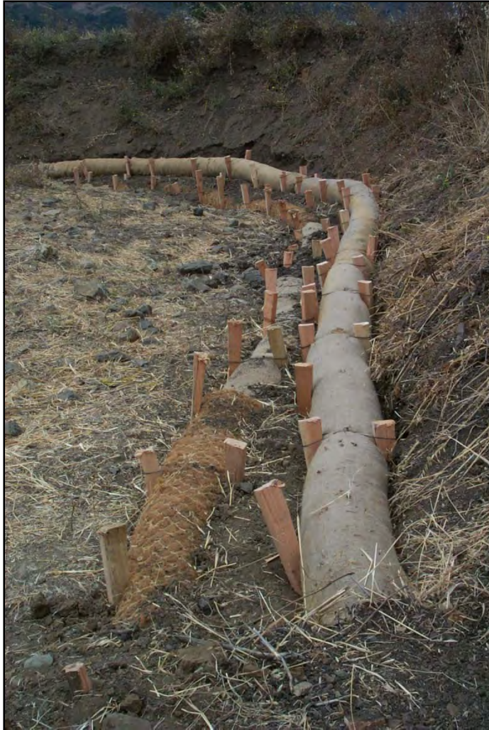
Figure 51. Installed coir logs.
