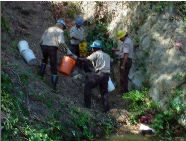
Figure 72. Corps hauling rock & soil out of site by hand.
