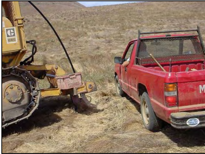
Figure 112. Rip shank and pipe feeder.
