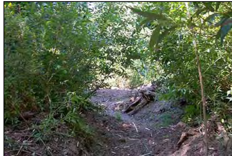
Figure 59. Channel opened up after CCC crews cleared debris
