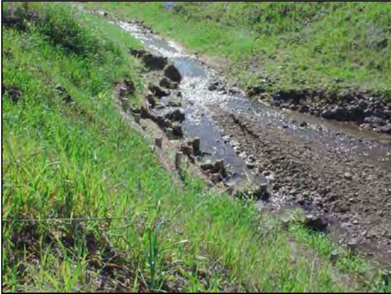
Figure 54. Grasses on bank behind coir logs.
