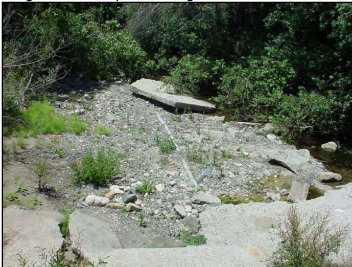
Figure 40. Concrete debris before removal.
