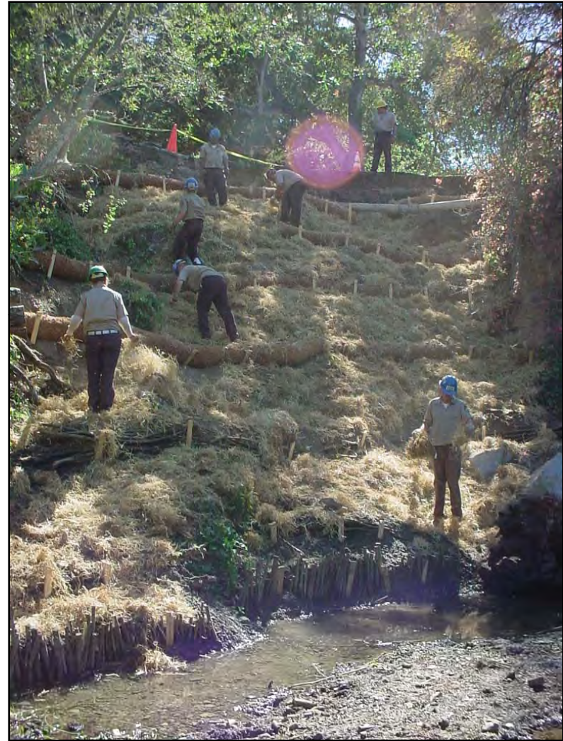
Figure 79. Straw applied for erosion protection being secured by CCC crews.
