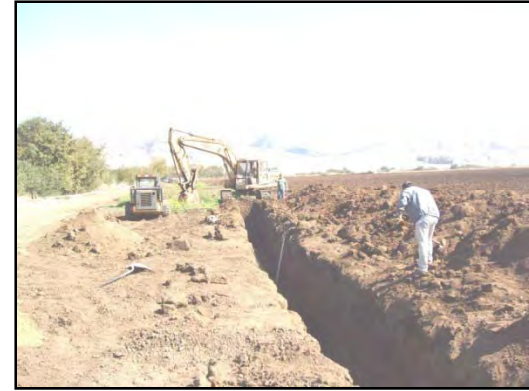
Figure 136. Installation by excavator.
