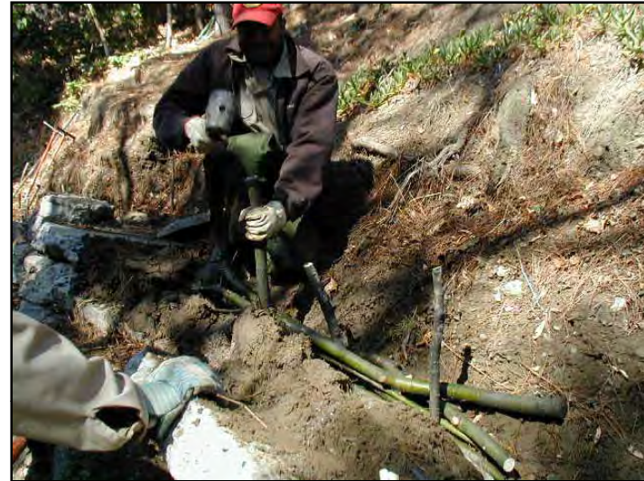
Figure 10. CCC crew planting willow stakes.
