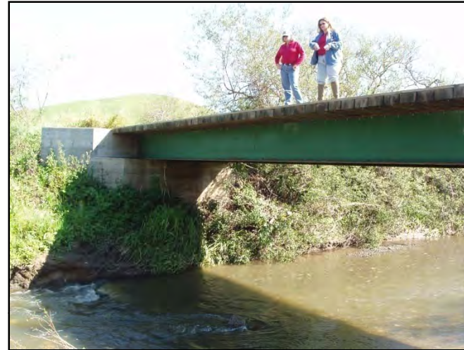
Figure 39. Cheryl Zelus admiring the completed bridge.
