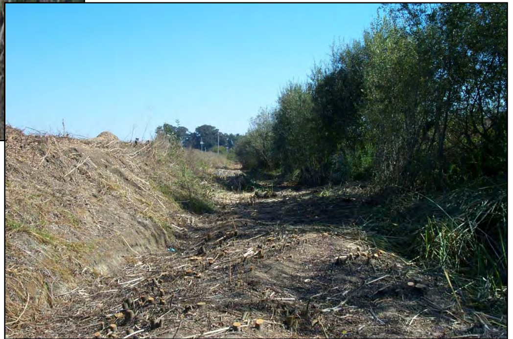
Figure 81. After pruning of willow in the center of the channel. Re-vegetation planting took place the following winter on the north side of channel.
