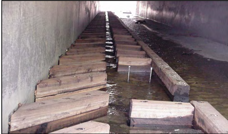
Figure 86. Dysfunctional baffles.
