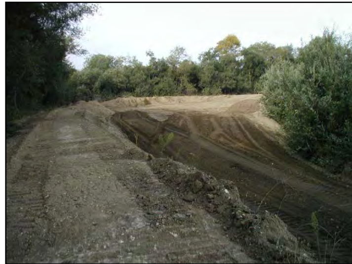
Figure 8. View of scraper path.
