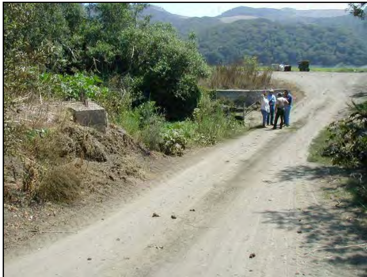
Figure 36. Partially completed abutments.
