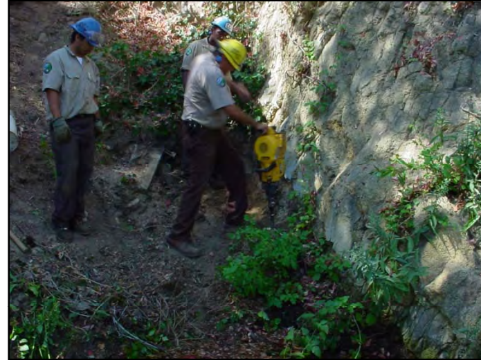
Figure 71. CCC hand digging and jack-hammering rock & soil out of site .
