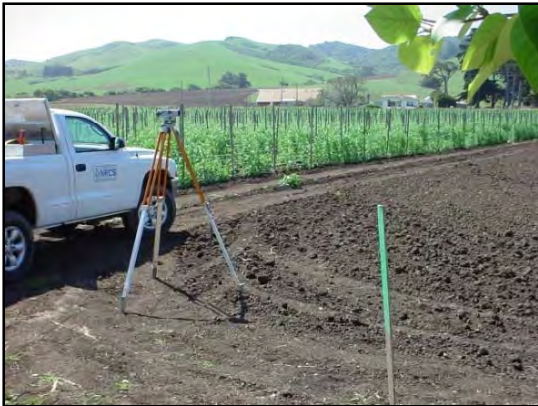
Figure 137. The pipeline was surveyed.
