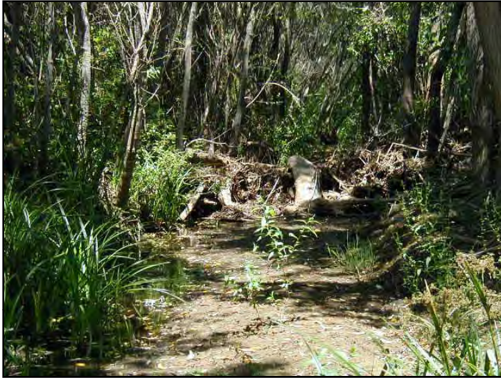
Figure 60. Debris jam in Los Osos Creek
