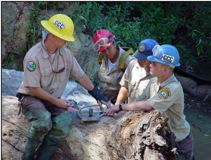
Figure 76. Corps members installing cabled boulders and root wad.
