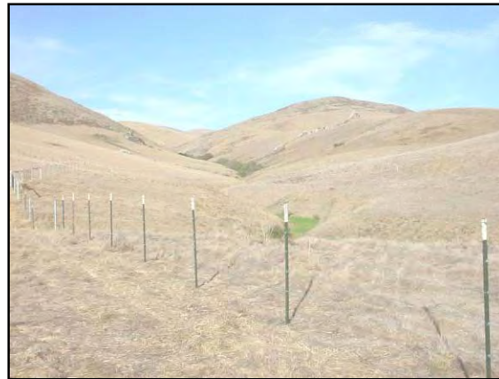
Figure 120. Installed fence along tributary.
