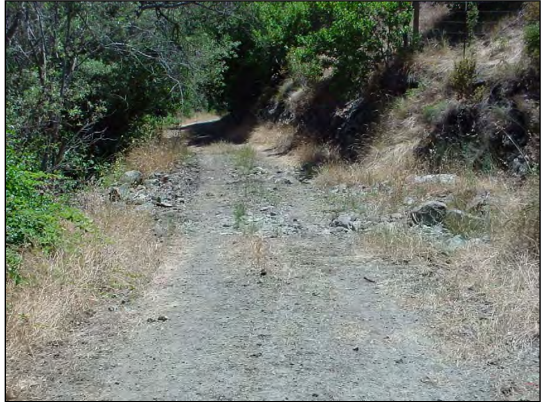
Figure 108. View of culvert after it was replaced with armored crossing.
