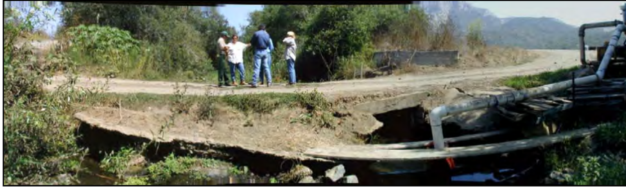
Figure 35. Existing Arizona stream crossing that was removed.
