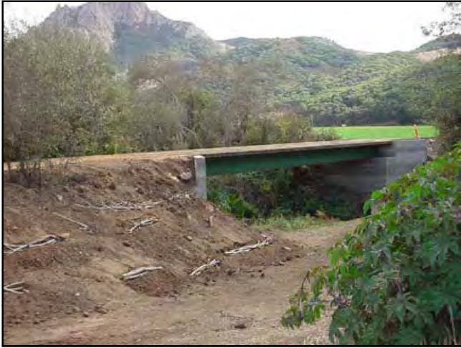
Figure 38. Completed bridge and bank stabilization.
