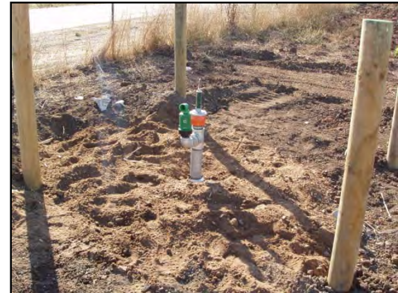
Figure 139. New combination air vent/Air release valve and a pressure relief valve.
