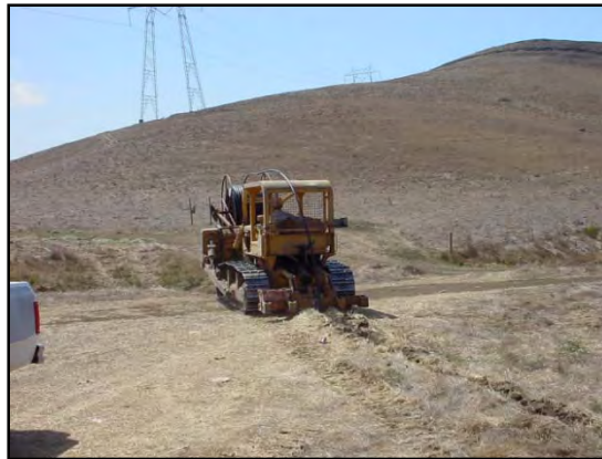
Figure 97. Low impact installation of pipeline.
