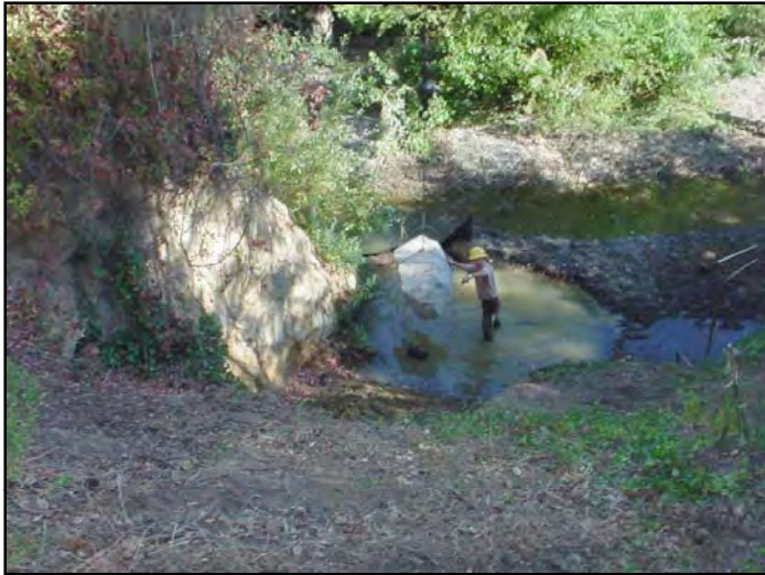
Figure 74. Boulders were craned in and guided into place by CCC.
