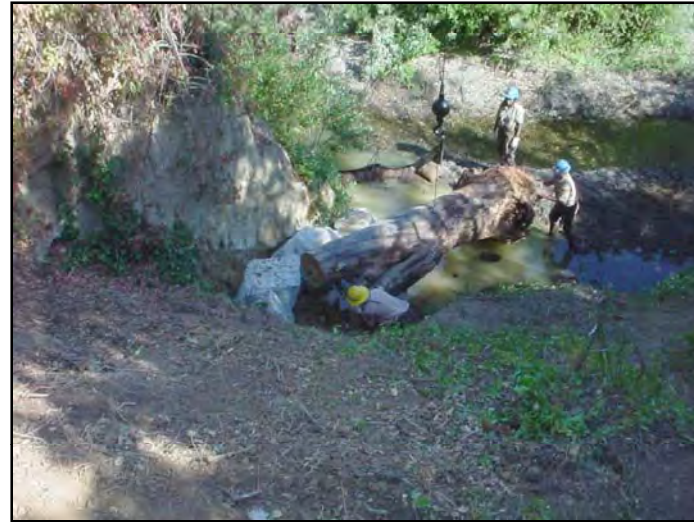
Figure 75. Corps members installing craned in root wad.
