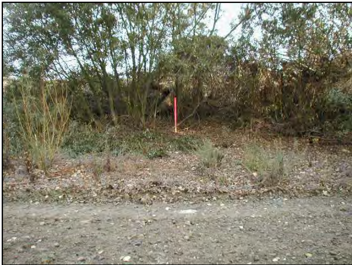
Figure 7. Cut stakes were placed to direct scraper.
