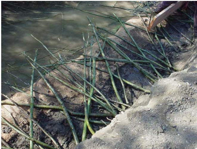
Figs. 13 & 14. Willow as it is laid into structure and covered with soil. Jute covers all exposed soil
