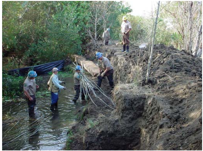
Fig 12. CCC crews excavated the bank by hand and laid in the willow.
