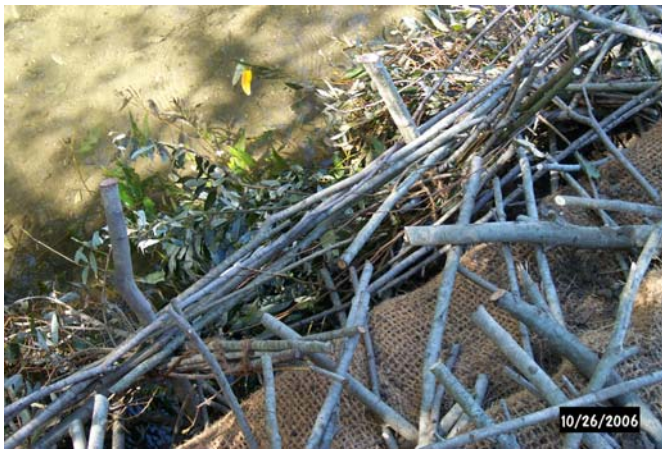
Fig 17. Recently harvested willow laid into project after watering.
