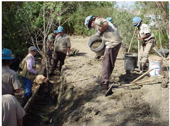
Figs. 13 & 14. Willow as it is laid into structure and covered with soil. Jute covers all exposed soil
