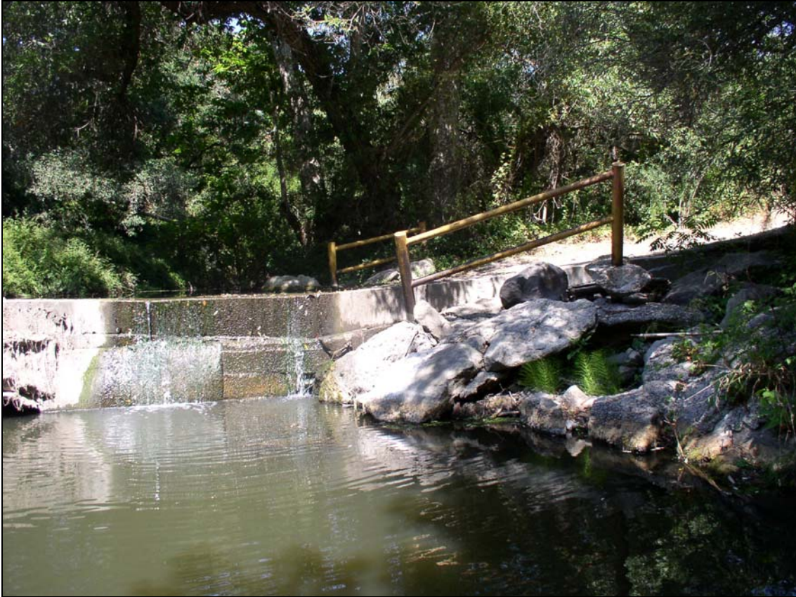
FIGURE 3.5 PISMO CREEK FISH BARRIER AT ARIZONA CROSSING
