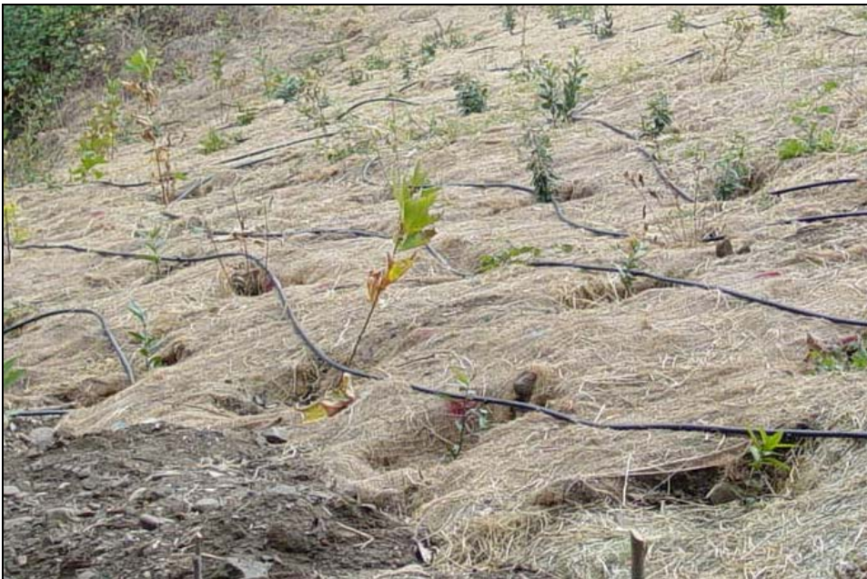
FIGURE 4.1 BANK STABILIZATION PROJECT ON WEST CORRAL DE PIEDRA CREEK
